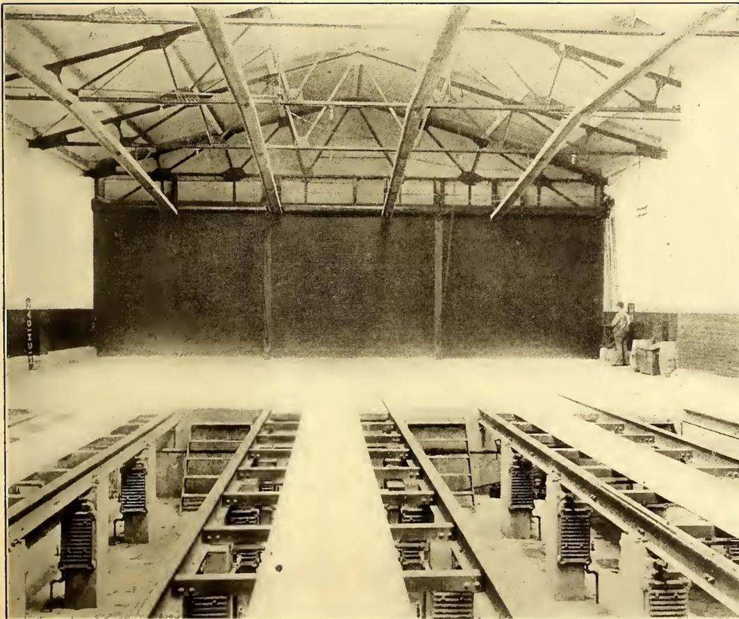
ROLLING DOOR AT THE REAR END OF THE CAR HOUSE, SHOWING ALSO DETAILS OF PIT CONSTRUCTION
