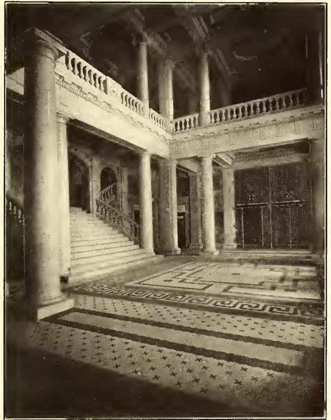
INTERIOR OF MAIN ENTRANCE TO THE BUILDING
