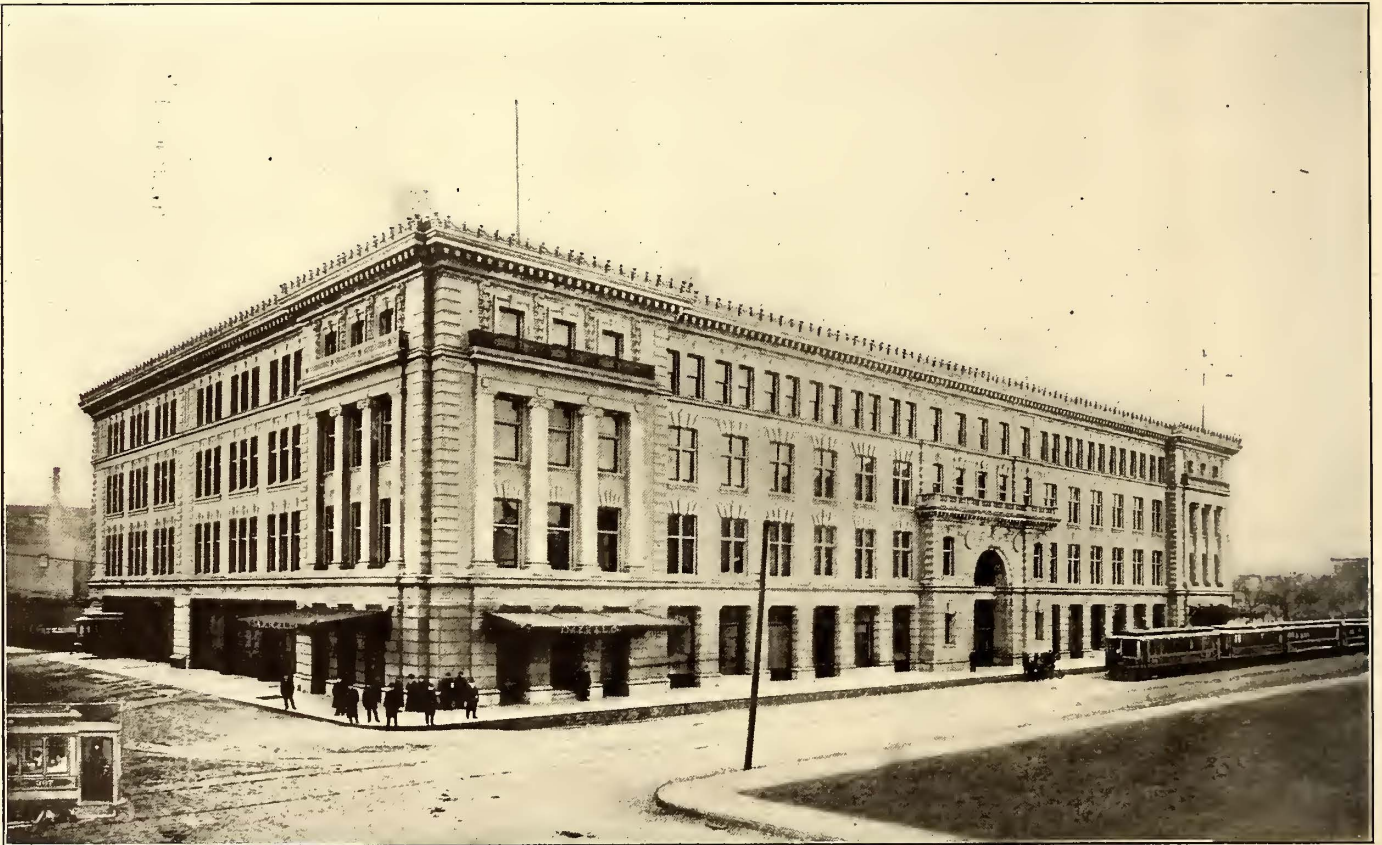
THE RECENTLY COMPLETED PUBLIC SERVICE BUILDING OF THE MILWAUKEE ELECTRIC RAILWAY & LIGHT COMPANY, AT MILWAUKEE
