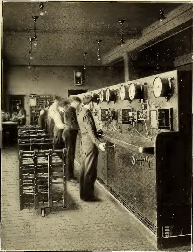
MOTOR-TESTING SIDE OF TEST BOARD IN TESTING ROOM
