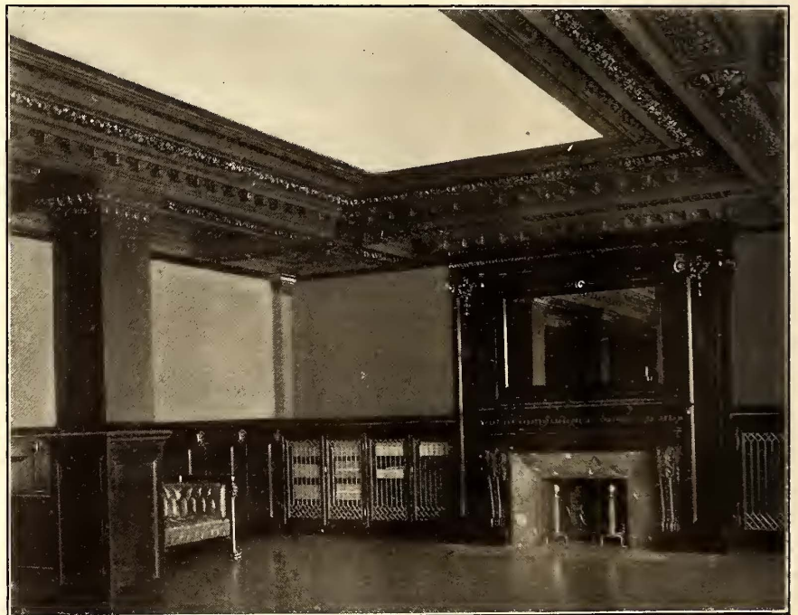
A CORNER IN THE DIRECTORS' ROOM, SHOWING THE RICH CARVINGS, ORNAMENTAL FIRE-PLACE, MANTEL, ETC.
