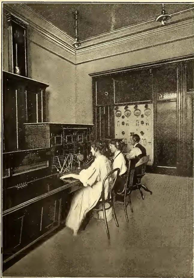
TELEPHONE ROOM, SHOWING DESPATCHERS' BOARD AND CENTRAL EXCHANGE FOR BUILDING
