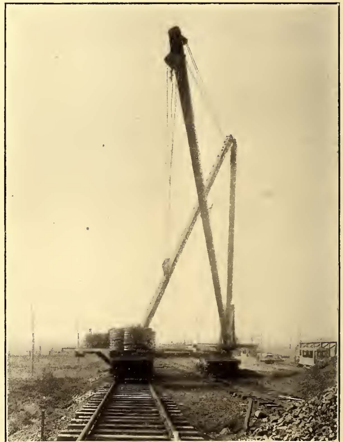
HOME-MADE TRAVELING DERRICK IN CLEVELAND
