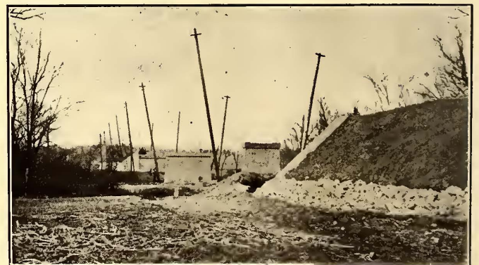
FIG. 2.—CONCRETE BUTTRESSES AND PIERS FOR STEEL STRUCTURES OVER CENTER CREEK
