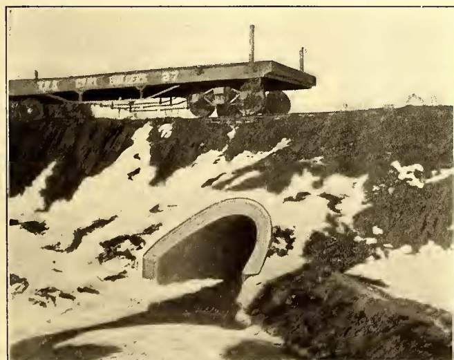
FIG. 3.—HORSESHOE ARCH ON THE INDIANAPOLIS & NORTH-WESTERN RAILWAY
