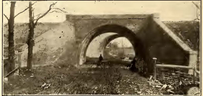
FIG. 7.—OVERHEAD CROSSING ON THE LIMA & TOLEDO RAILWAY
