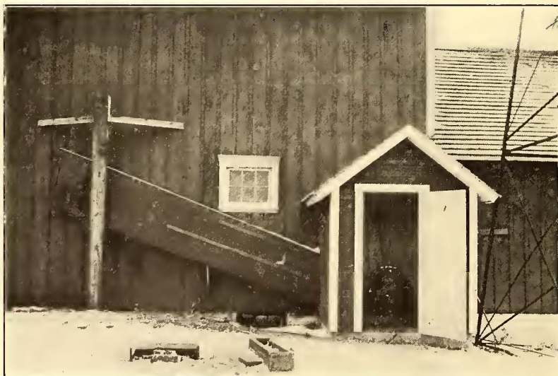
MOTOR HOUSE IN WHICH A 15-HP MOTOR IS INSTALLED FOR OPERATING FARM MACHINERY
