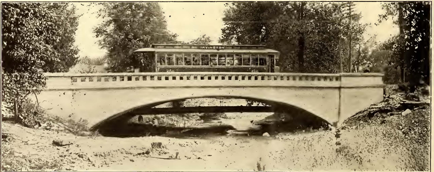
FIG. 8.—A 65-FT. CONCRETE ARCH ON EAST WASHINGTON STREET, INDIANAPOLIS
