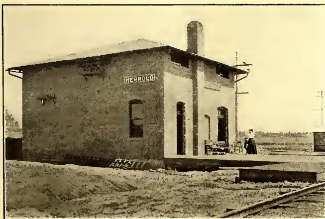
PRESENT SUB-STATION BUILDING AND STATION AT HERROLD
