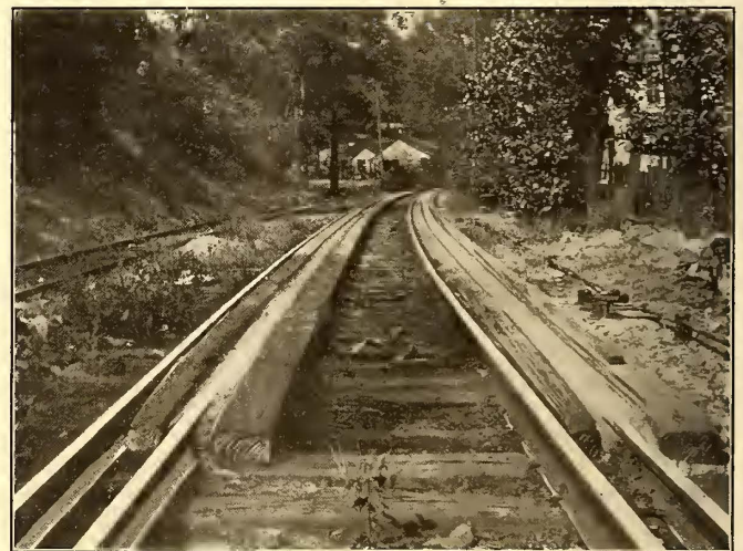
SANDED TRACK AT SIDE OF MAIN LINE TRACKS FOR STOPPING RUN-AWAY CARS—NEW JERSEY & HUDSON RIVER RAILWAY
