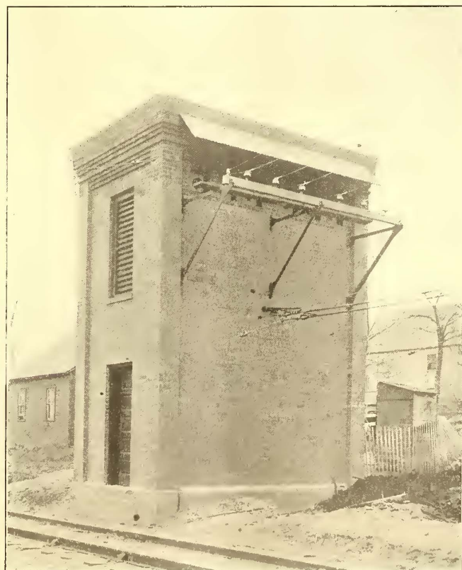
BRICK CABLE HOUSE NEAR CITY LIMITS
