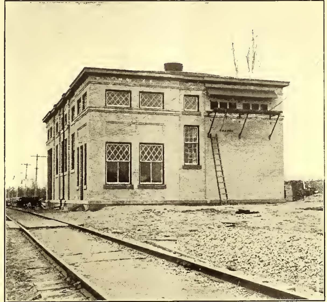
THE EXCELSIOR SUB-STATION
