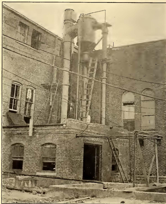
CONDENSER INSTALLATION FOR VERTICAL TURBINE
