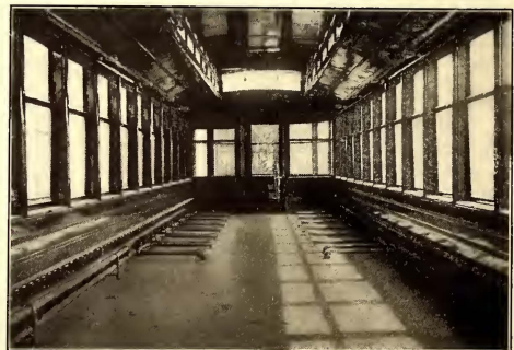
INTERIOR OF DOUBLE-DECK CAR, SHOWING THE SIDE GIRDERS OF THE STEEL BOTTOM FRAMING
