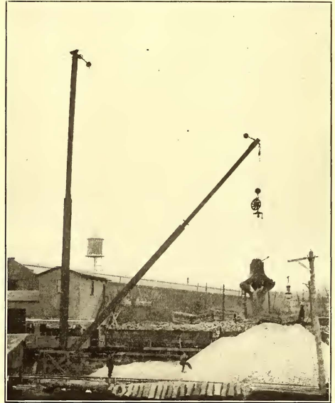
GRAB-BUCKET DUMPING LOAD OF DIRT
