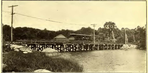
A LONG TRESTLE NEAR NOANK, ON THE LINE OF THE GROTON & STONINGTON STREET RAILWAY COMPANY
