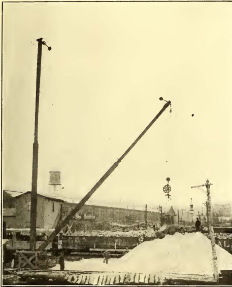
GRAB-BUCKET OPENING TO TAKE LOAD OF MATERIAL
