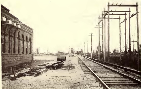
LINE ANCHORAGE AT POWER STATION, SCIOTO VALLEY
