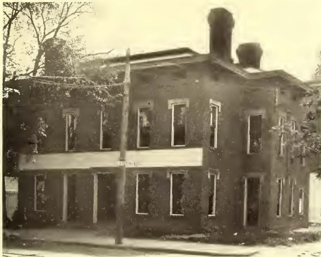
TERMINAL STATION AT MARION, COLUMBUS, DELAWARE & MARION
