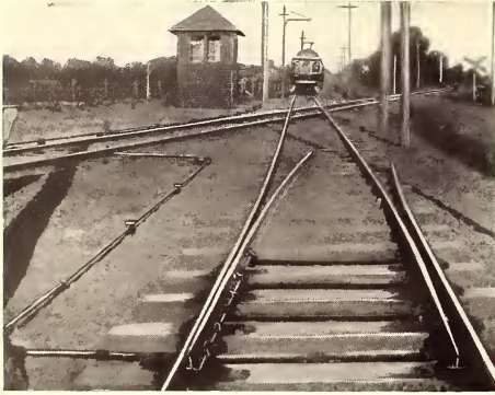
INTERLOCKER, WESTERN OHIO
