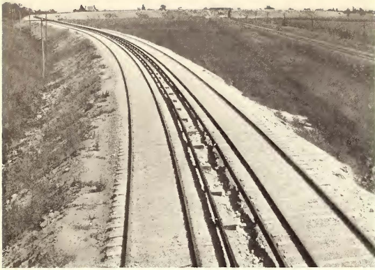
THE "BIG FILL" AT OVERCROSSING WITH H. V. RAILWAY, SCIOTO VALLEY
