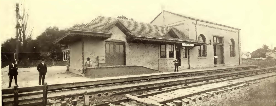
COMBINATION FREIGHT, PASSENGER AND SUB-STATION AT KINGSTON, SCIOTO VALLEY
