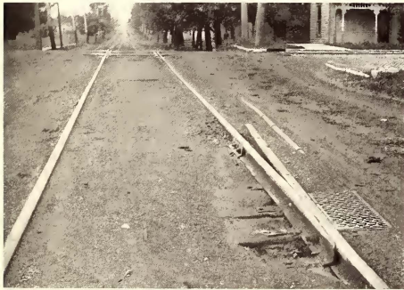
TYPE OF DERAIL, INDIANAPOLIS & NORTHWESTERN
