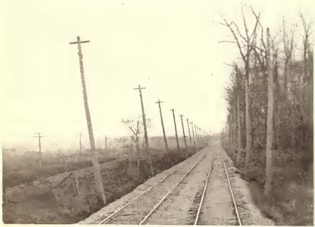
DOUBLE-TRACK CONSTRUCTION, DAYTON & TROY
