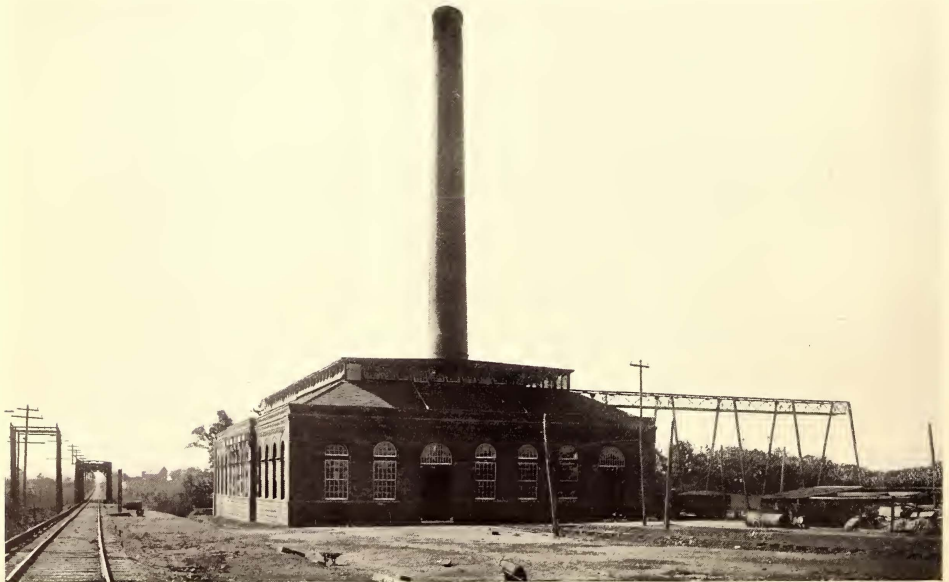
EXTERIOR POWER STATION, SCIOTO VALLEY
