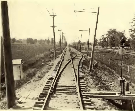
SWITCH STAND AND TELEPHONE BOOTH, TYPICAL TURNOUT, COLUMBUS, DELAWARE & MARION
