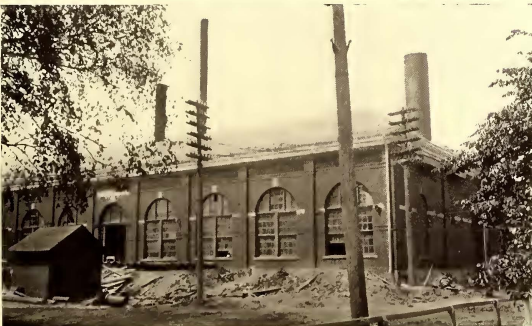
POWER STATION AT FINDLAY, TOLEDO URBAN & INTERURBAN
