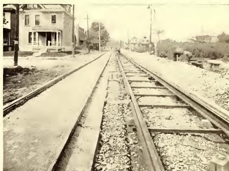
CONCRETE GIRDER CONSTRUCTION IN COLUMBUS. TO BE PAVED WITH BRICK. ONE TRACK CONCRETED. MATERIAL BEING DELIVERED IN OTHER TRACK
