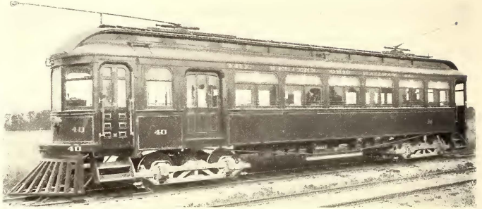
LIMITED CAR, WESTERN OHIO RAILWAY (LENGTHENED IN OWN SHOPS)
