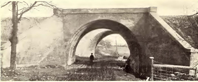
TYPE OF CONCRETE BRIDGE USED BY SEVERAL INTERURBAN ROADS IN OHIO
