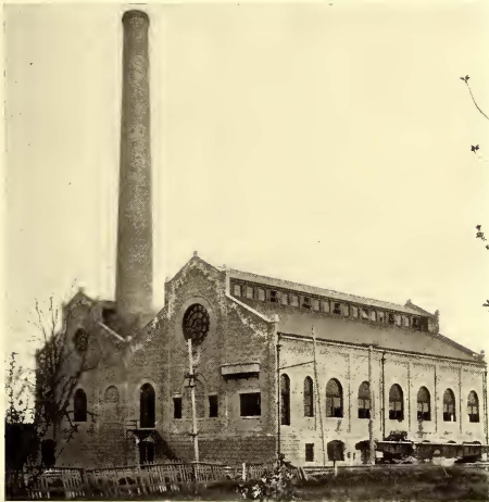
POWER STATION AT HEBRON, COLUMBUS, BUCKEYE & NEWARK
