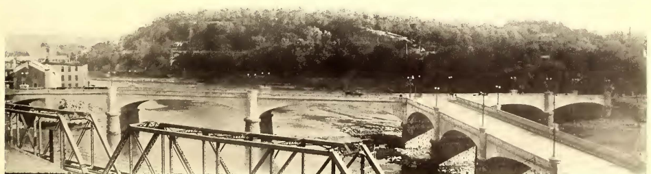
THE FAMOUS Y CONCRETE BRIDGE AT ZANESVILLE, OHIO
