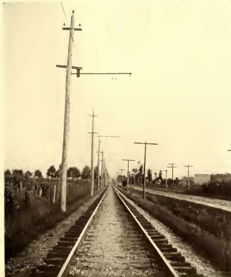
TYPICAL CONSTRUCTION, INDIANAPOLIS, COLUMBUS & SOUTHERN TRACTION
