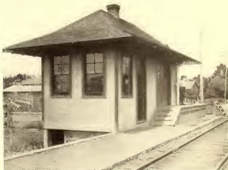
FREIGHT AND PASSENGER STATION AT LOCKBOURNE, SCIOTO VALLEY
