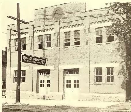
AUTOMOBILE STORAGE BATTERY STATION MAINTAINED BY COLUMBUS RAILWAY & LIGHT COMPANY
