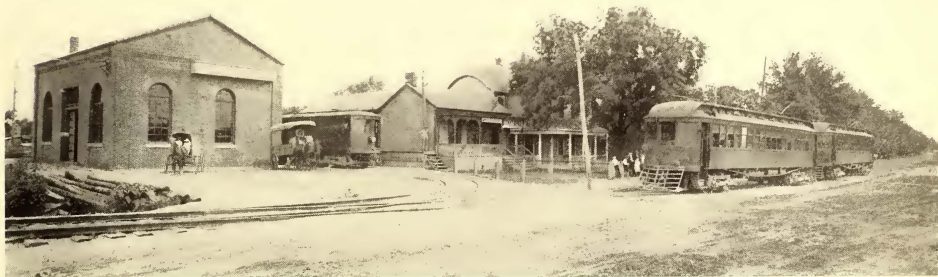
SUB-STATION AND TEMPORARY FREIGHT AND PASSENGER STATION AT CHILLICOTHE, SCIOTO VALLEY
