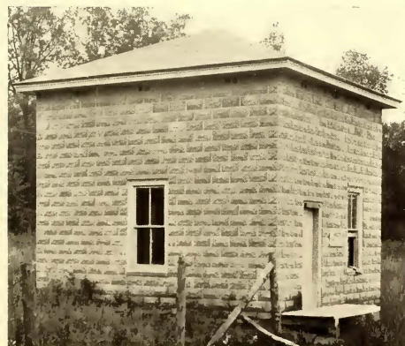
CONCRETE BLOCK SUB-STATION, TOLEDO & INDIANA
