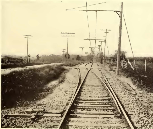
TYPICAL SWITCH, WESTERN OHIO
