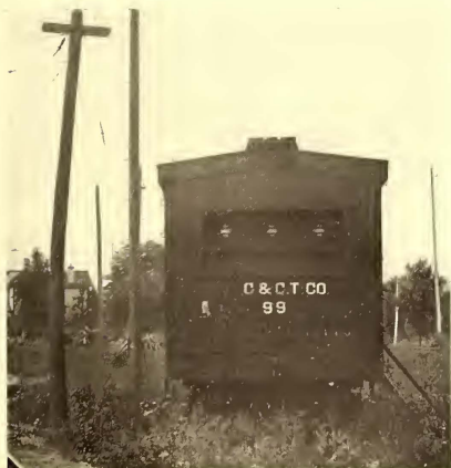
PORTABLE SUB-STATION, CINCINNATI & COLUMBUS
