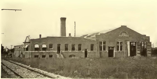
CAR HOUSE, SHOPS AND OPERATING HEADQUARTERS, WESTERN OHIO RAILWAY
