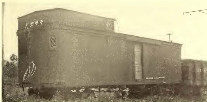
PORTABLE SUB-STATION, TOLEDO & WESTERN RAILWAY
