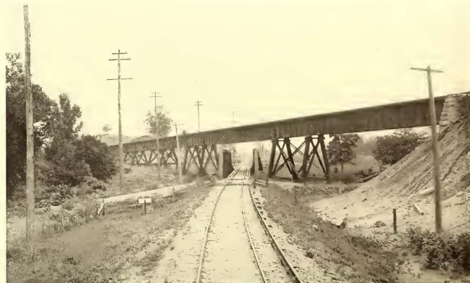
UNDERCROSSING WITH THE N. & W. RAILWAY AT KINNIKINNICK, SCIOTO VALLEY
