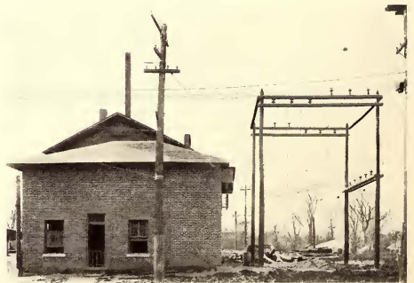
PROSPECT SUB-STATION, COLUMBUS, DELAWARE & MARION
