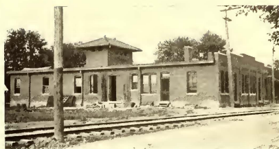
SUB-STATION AND BATTERY HOUSE, DAYTON & MUNCIE
