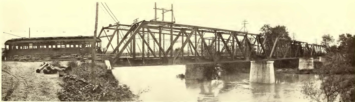
STEEL BRIDGE OVER SCIOTO RIVER AT ENTRANCE TO CHILLICOTHE, SCIOTO VALLEY TRACTION COMPANY
