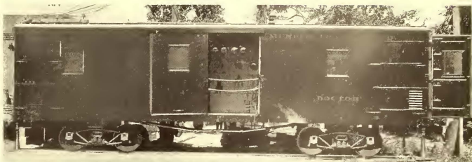
PORTABLE SUB-STATION, DAYTON & MUNCIE
