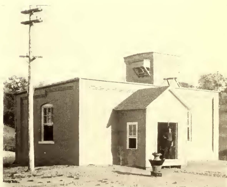
SUB-STATION, COLUMBUS, NEWARK & ZANESVILLE
