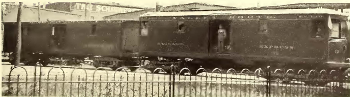
MOTOR AND TRAILER FOR EXPRESS AND FREIGHT SERVICE, SCIO VALLEY TRACTION
