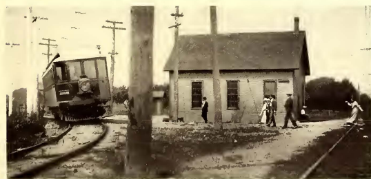
JUNCTION STATION, LAKE SHORE ELECTRIC
