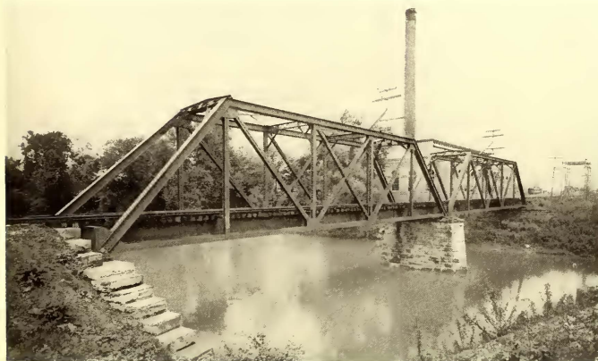
VIEW AT BIG WALNUT CREEK, SHOWING STANDARD BRIDGE CONSTRUCTION, POWER HOUSE IN BACKGROUND—SCIOTO VALLEY
