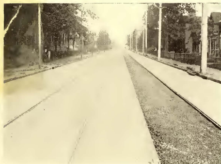
CONCRETE GIRDER CONSTRUCTION IN COLUMBUS. ASPHALT PAVEMENT COMPLETED, EXCEPT TOP COAT IN ONE TRACK
