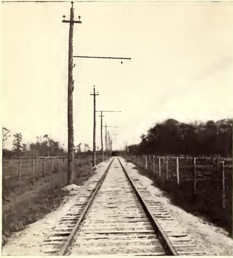
TYPICAL CONSTRUCTION, TOLEDO, PT. CLINTON & LAKESIDE
