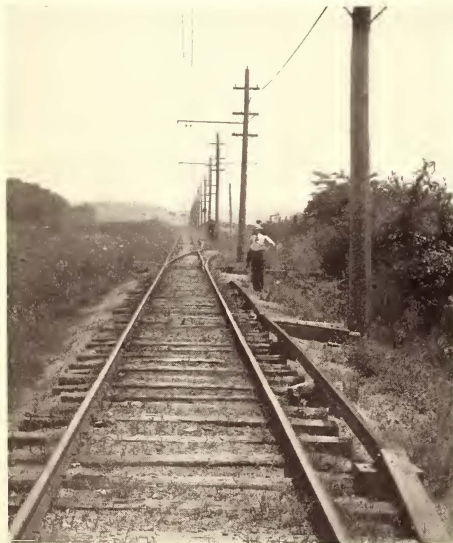
THIRD RAIL FOR OPERATING SIGNALS AT TURNOUTS, COLUMBUS, NEWARK & ZANESVILLE
