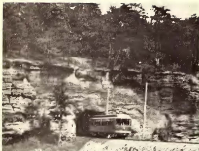
THE TUNNEL ON THE COLUMBUS, NEWARK & ZANESVILLE LINE
