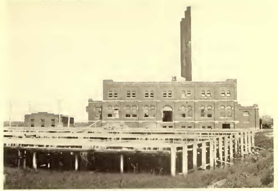
POWER STATION, BATTERY HOUSE AND WATER-COOLING TRAYS, DAYTON & MUNCIE
