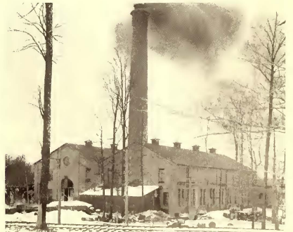
POWER STATION AT ELYRIA, CLEVELAND & SOUTHWESTERN
