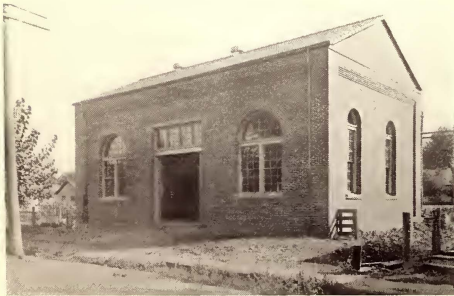
SUB-STATION BUILDING, SCIOTO VALLEY
