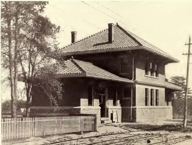
FORESTVILLE COMBINED PASSENGER AND SUB-STATION, INTERURBAN RAILWAY & TERMINAL COMPANY, CINCINNATI
