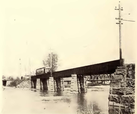
OLENTANGY RIVER BRIDGE, COLUMBUS, DELAWARE & MARION
