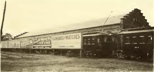
STORING CARS OUTDOORS, PROTECTING FENCE TO SHIELD THEM, PAID FOR BY ADVERTISING, STARK ELECTRIC
