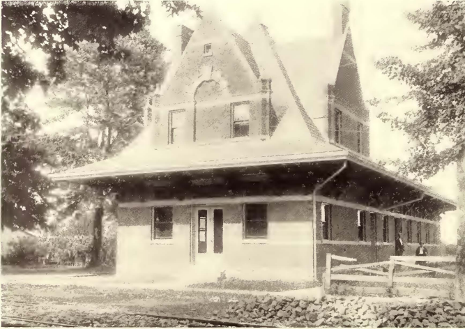
AMELIA SUB-STATION AND WAITING ROOM, INTERURBAN RAILWAY & TERMINAL COMPANY, CINCINNATI
