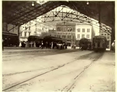
TRAIN SHED, INTERURBAN UNION STATION, INDIANAPOLIS
