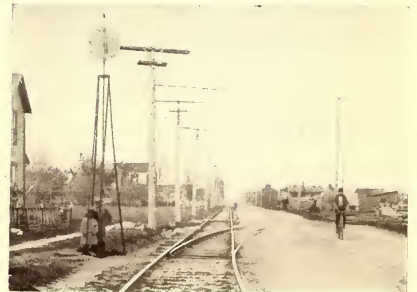
SWITCH STAND AT TURNOUTS, COLUMBUS, LONDON & SPRINGFIELD
