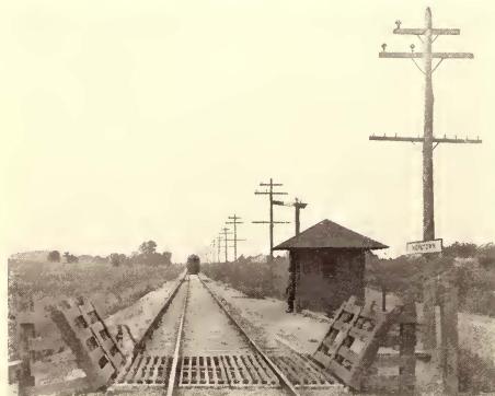
STANDARD OPEN WAITING STATION AND TRAIN-SIGNALING DEVICE, SCIOTO VALLEY
