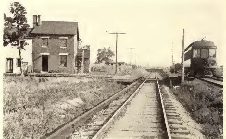
ORETZ JUNCTION, THE JUNCTION POINT OF LANCASTER AND CHILlicothe DIVISIONS. THE PASSENGER STATION PLATFORM EXTENDS OVER THIRD RAIL—SCIOTO VALLEY
