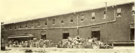
SIDE VIEW, INTERURBAN FREIGHT STATION AT INDIANAPOLIS
