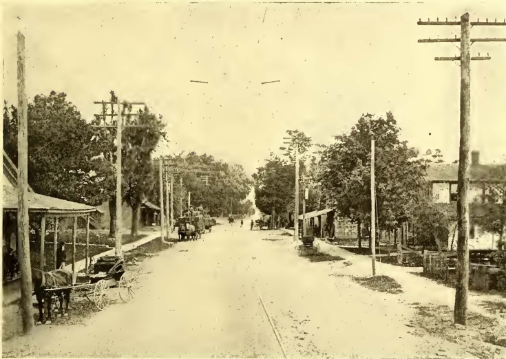
FIG. 13.—SPAN CATENARY CONSTRUCTION USED THROUGH TOWNS
