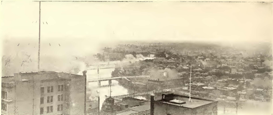
SCIOTO RIVER AND BIRD'S-EYE VIEW OF COLUMBUS, LOOKING SOUTH, WIRELESS TELEGRAPH STATION SHOWN AT LEFT
