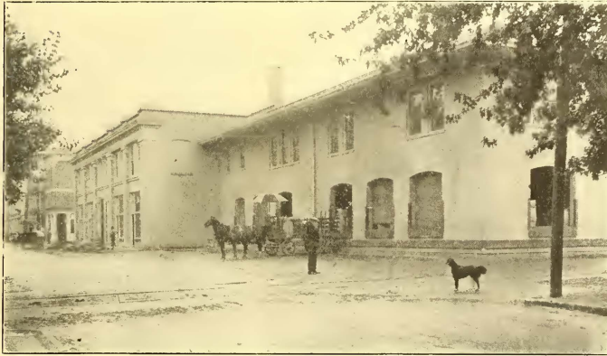
SOUTH MULBERRY STREET FRONT OF TERMINAL BUILDING AND FREIGHT HOUSE
