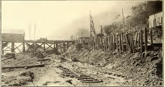
WORK IN PREPARING NEW ROADWAY ON CUT-OFF
