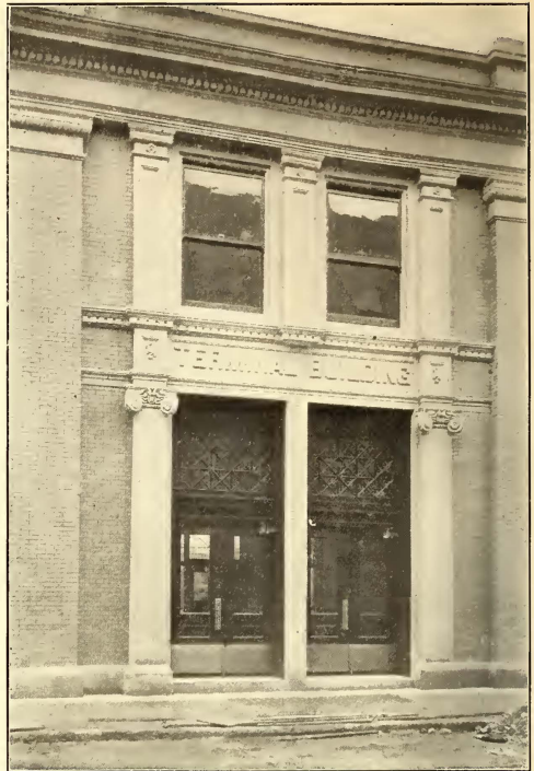
ENTRANCE TO TERMINAL BUILDING ON SOUTH MULBERRY STREET
