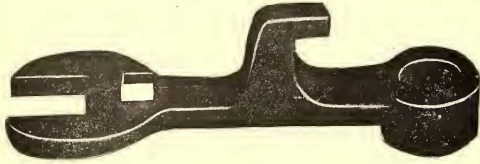
FIG. 1.—COMBINATION REVERSE WRENCH
