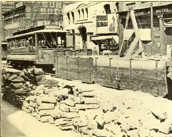
COVER CAR USED FOR BLASTING IN OLIVE STREET
