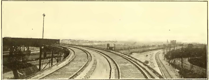
ARRANGEMENT OF CROSSING OF THE PHILADELPHIA & READING AND THE PENNSYLVANIA RAILROAD TRACKS
