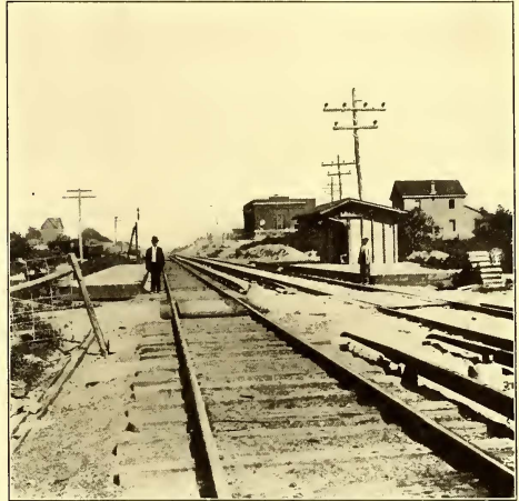
FIG. 21.—THIRD RAIL AND TRANSMISSION LINE
