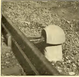
FIG. 32.—SINGLE THIRD-RAIL JUMPER
