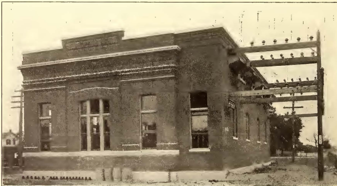
FIG. 16.—EXTERIOR OF GLASSBORO SUB-STATION
