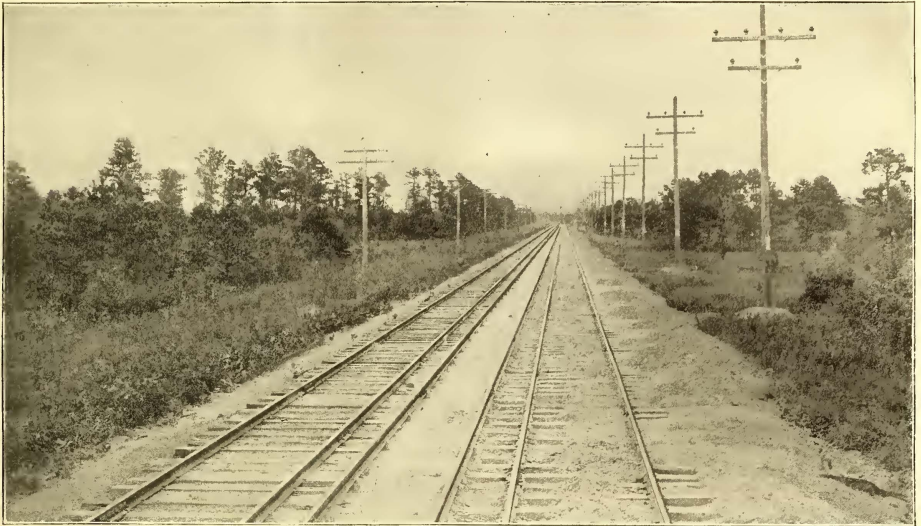
FIG. 23.—SECTION OF TRACK NEAR MIZPAH, N. J., SHOWING THIRD RAIL AND TRANSMISSION LINE
