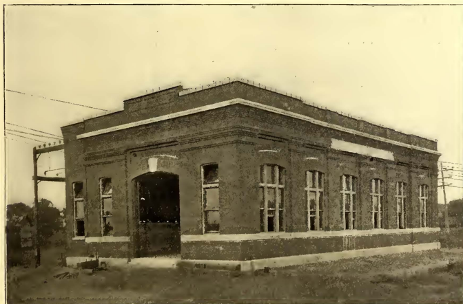
FIG. 17.—EXTERIOR OF NEWFIELD SUB-STATION
