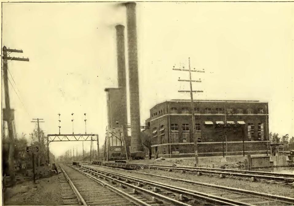
FIG. 3.—GENERAL VIEW OF WESTVILLE POWER STATION
