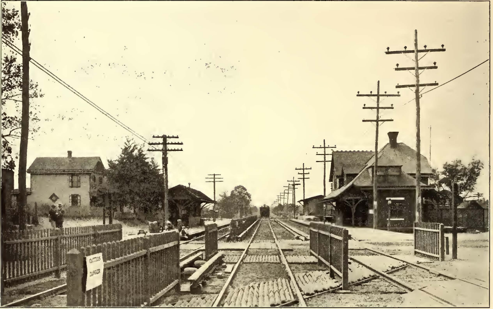
FIG. 22.—CATTLE GUARDS, JUMPERS, APPROACH BLOCKS AND THIRD-RAIL COVERING AT WESTVILLE
