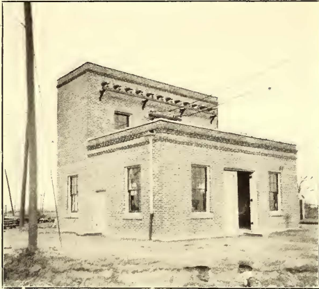
EXTERIOR OF SUB-STATION AT GOSHEN
