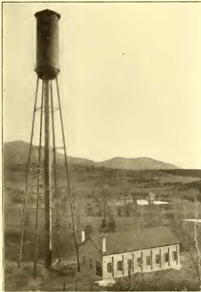
FIG. 2.—RUTLAND RAILWAY, LIGHT & POWER COMPANY'S POWER HOUSE
