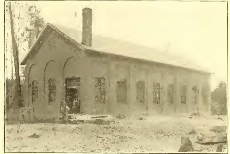
FIG. 3.—EXTERIOR OF POWER STATION
