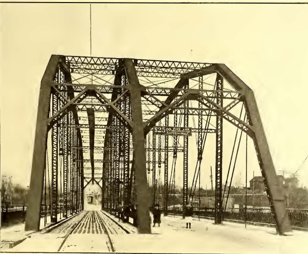
A RECONSTRUCTED HIGHWAY BRIDGE
