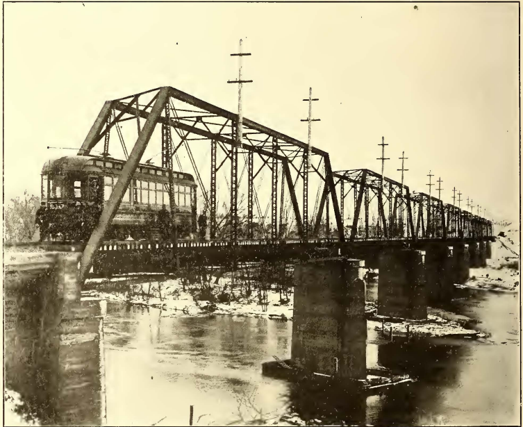
BRIDGE OF SOUTH BEND & SOUTHERN MICHIGAN RAILWAY, OVER ST. JOSEPH RIVER
