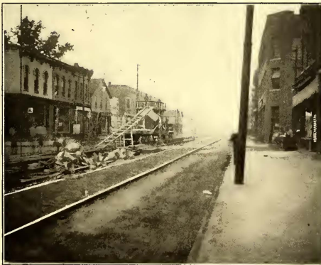
FIG. 12.—CONCRETE MIXER, SHOWING SLOPING TRACK TO THE PLATFORM ABOVE THE DRUM
