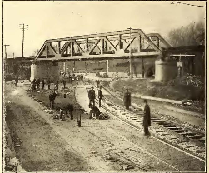
DOUBLE S CURVE UNDER BRIDGE, BEFORE AND AFTER STRAIGHTENING TRACK
