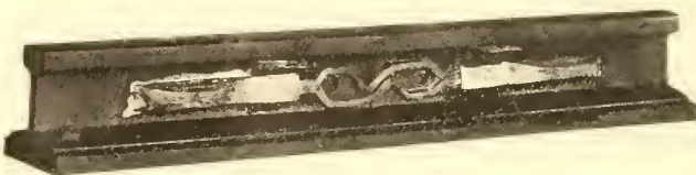
THE BOND IMMEDIATELY AFTER WELDING
