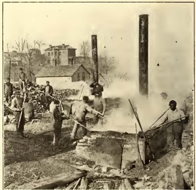
STIRRING THE ASPHALT DURING THE HEATING PROCESS
