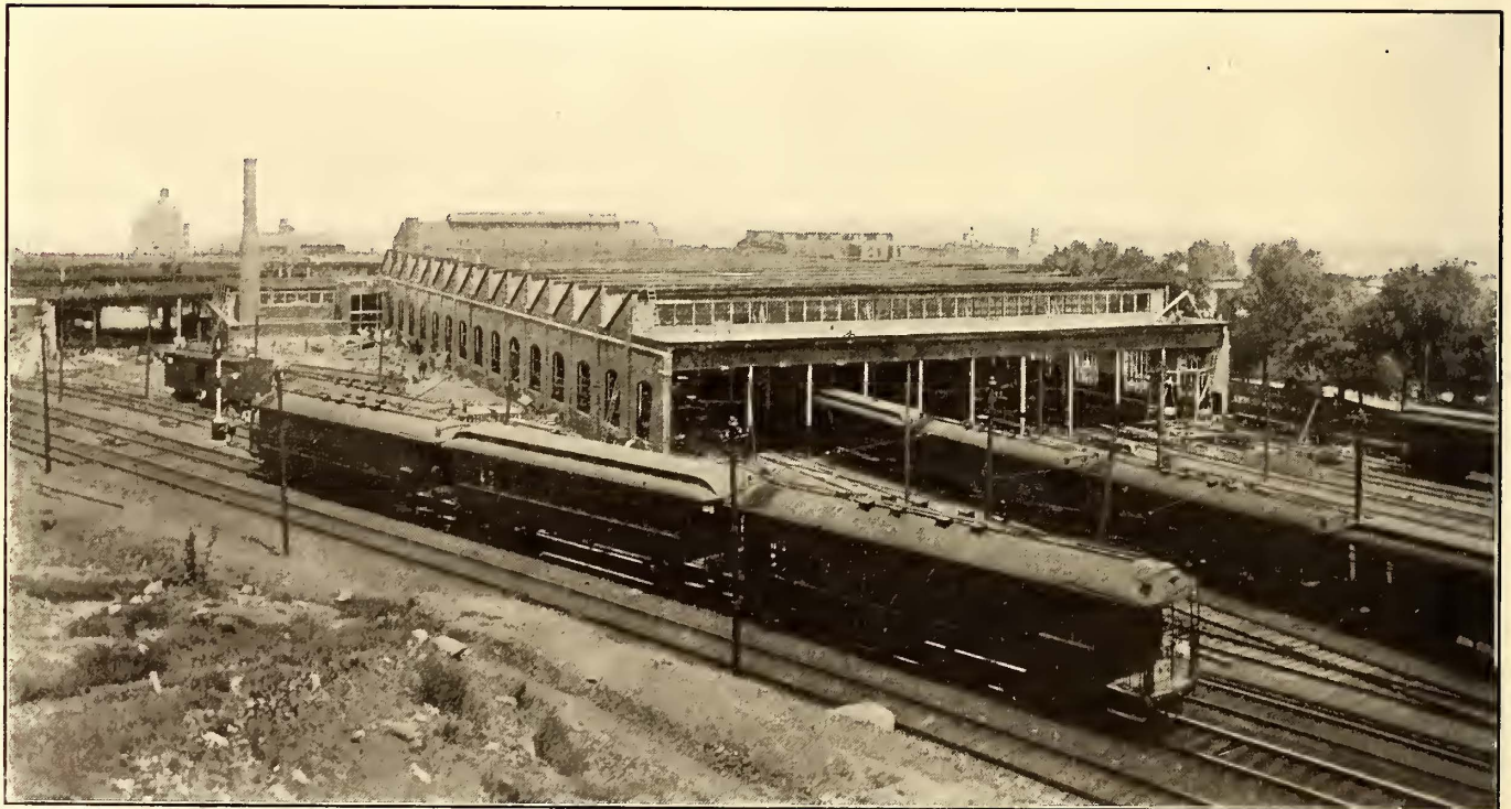
FIG. 2.—GENERAL VIEW OF THE THIRTY-SIXTH STREET INSPECTION PLANT, TAKEN FROM THE STORAGE YARD
