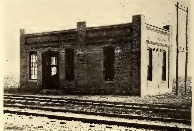
EXTERIOR OF THE BOONVILLE SUB-STATION
