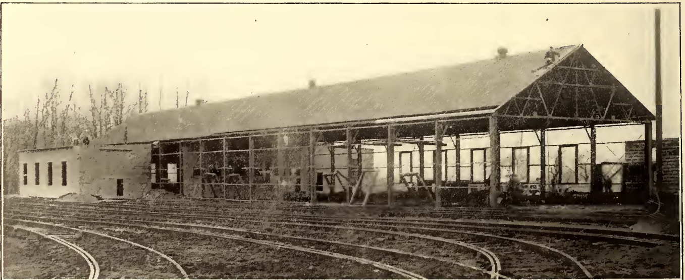
CAR HOUSE FRAMING AND ROOF NEARLY COMPLETED, ALSO SHOWING THE ADJOINING CAR-WASHING HOUSE
