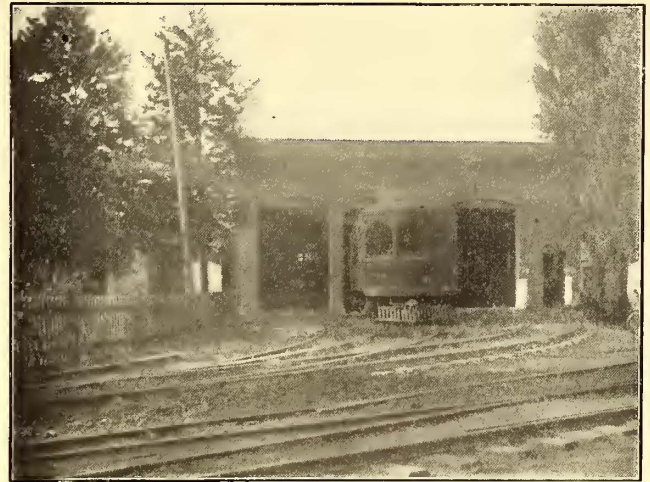
CAR HOUSE OF THE EVANSVILLE-BOONVILLE LINE
