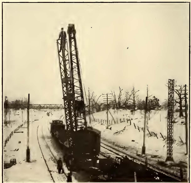
FIG. 6.—END VIEW OF CONSTRUCTION CRANE
