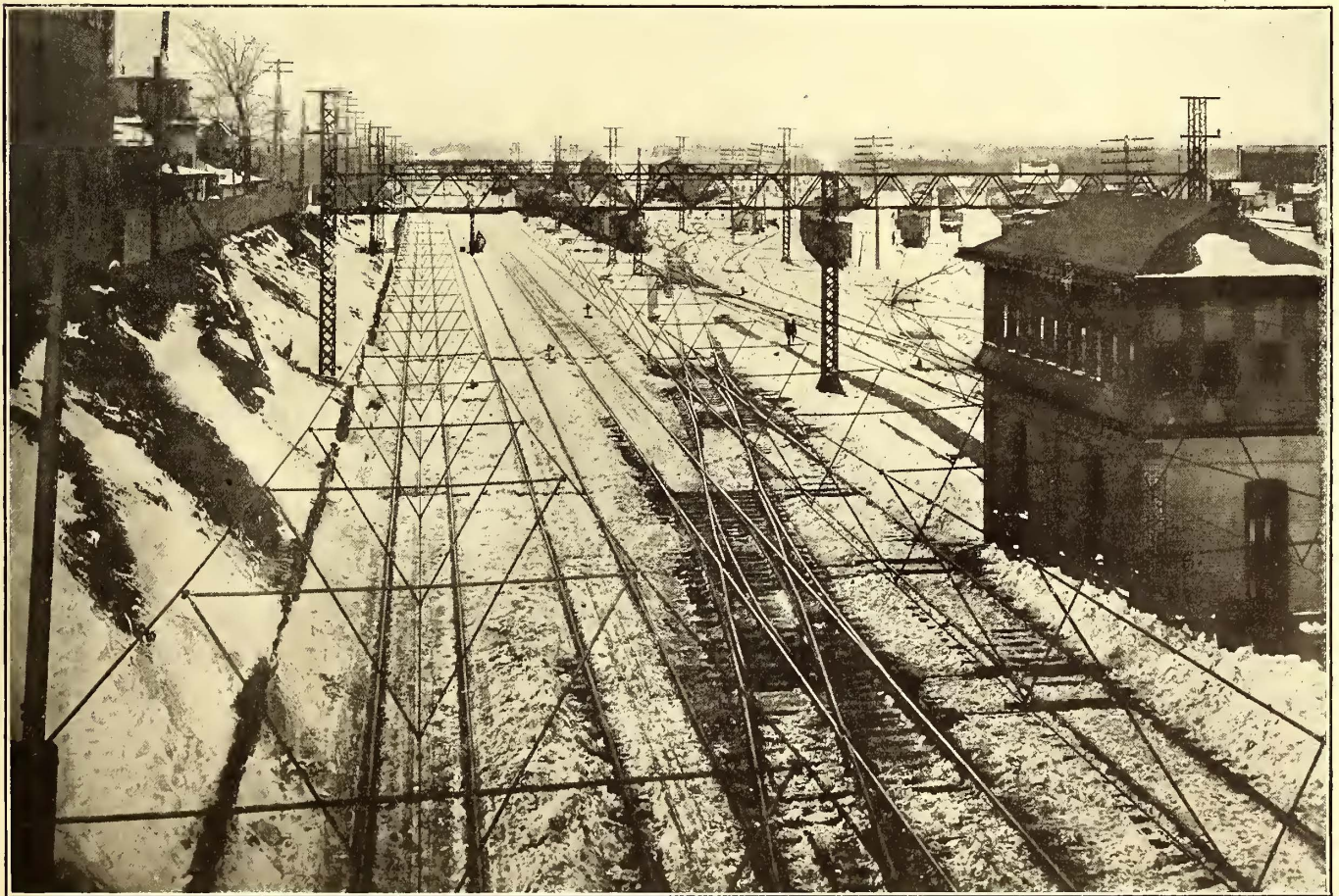
FIG. 2.—VIEW FROM THE NEW ROCHELLE ANCHOR BRIDGE NO. 72, LOOKING EAST
