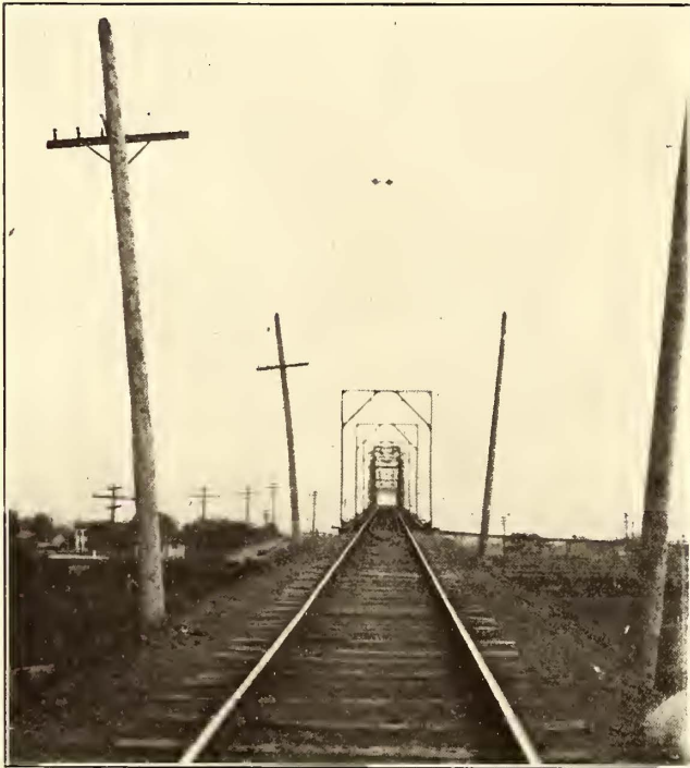
NORTH APPROACH OF THE EAST ST. LOUIS VIADUCT
