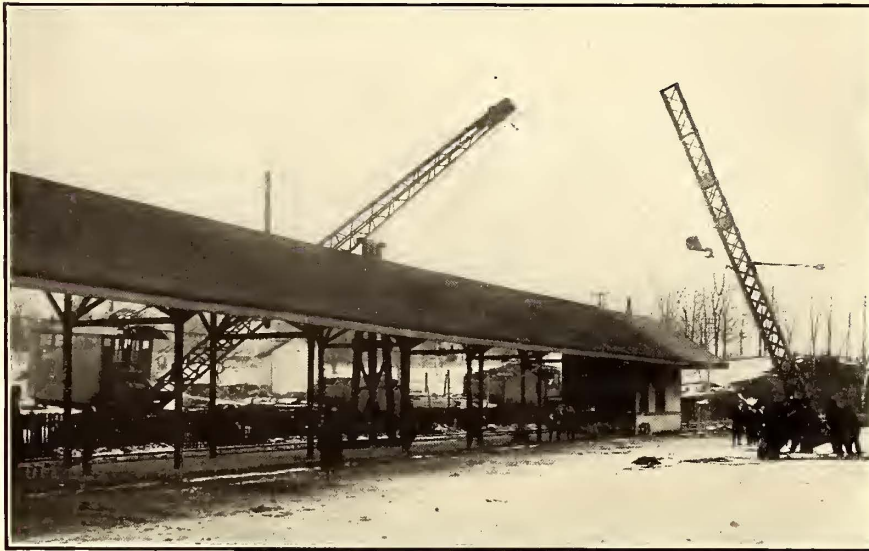
FIG. 5.—SETTING POLE IN PLACE AT RYE
