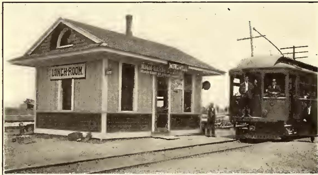
INTERURBAN STATION AT THE JUNCTION AT MITCHELL
