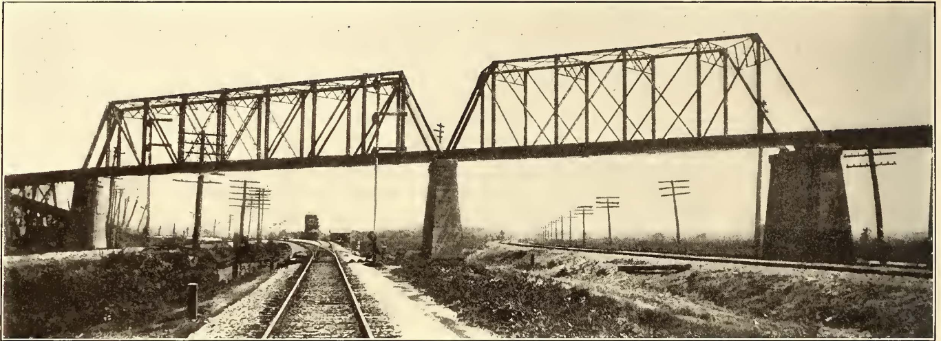
VIEW SHOWING ANGULARITY OF CROSSING TRACKS ON MITCHELL VIADUCT
