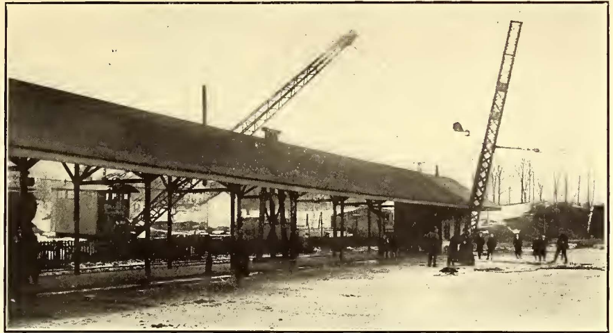
FIG. 4.—SETTING POLE IN PLACE AT RYE
