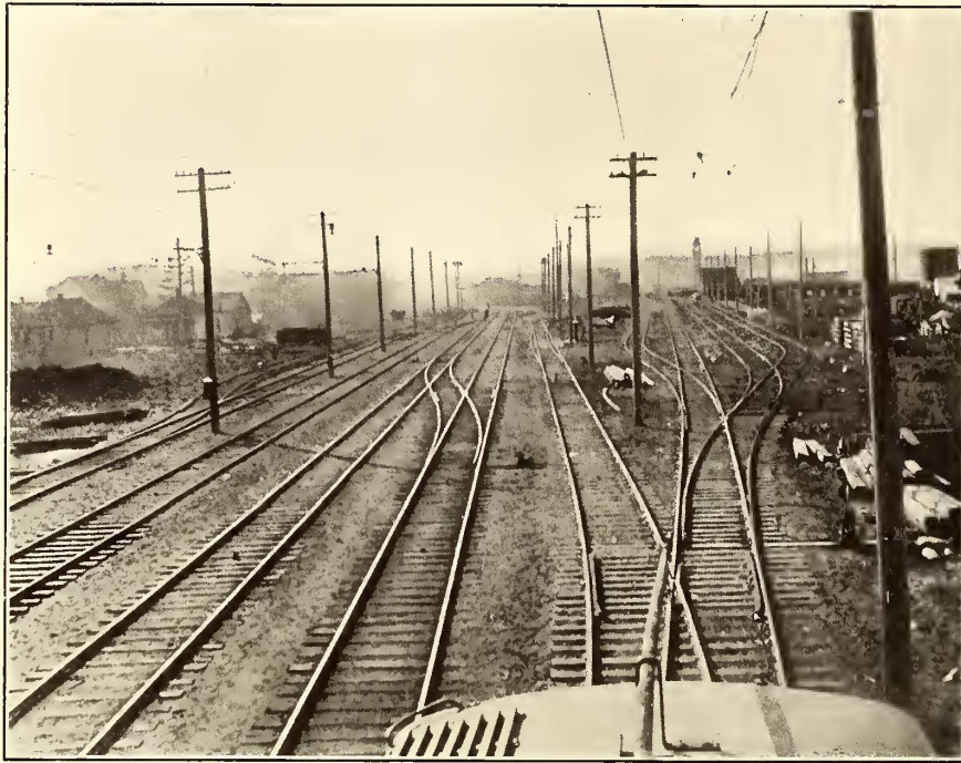
A PORTION OF THE FREIGHT YARDS OF THE INLAND EMPIRE SYSTEM AT SPOKANE. THESE YARDS ARE 300 FT. WIDE AND 2000 FT. LONG
