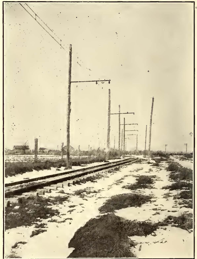
TROLLEY CONSTRUCTION ON CURVES, SHOWING "BRIDLE" IN THE FOREGROUND
