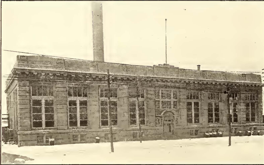
EXTERIOR OF CENTRAL PENNSYLVANIA TRACTION COMPANY'S POWER STATION, HARRISBURG, PA.
