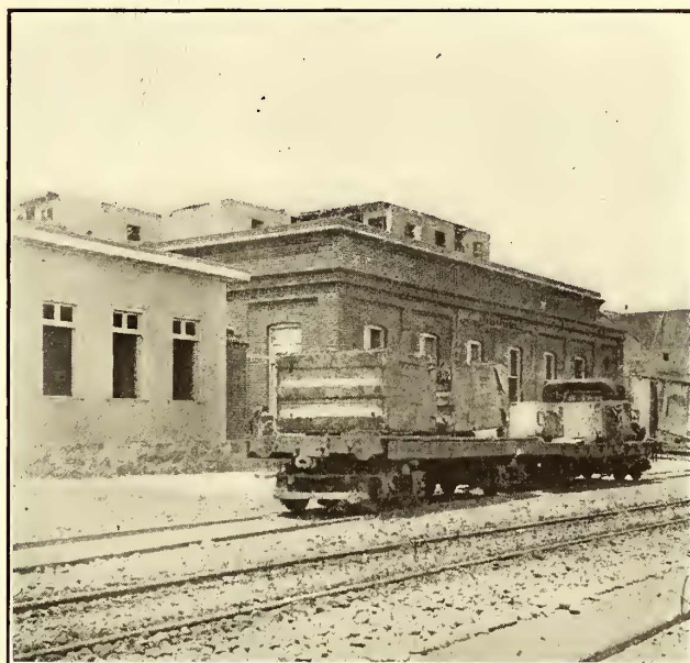
EXTERIOR VIEW OF THE SUB-STATION
