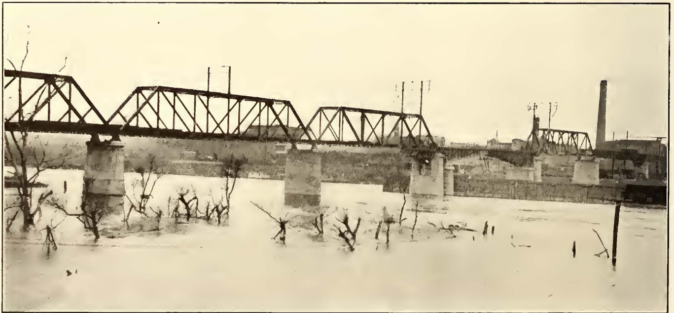
BASCULE BRIDGE OVER THE ILLINOIS RIVER AT PEORIA
