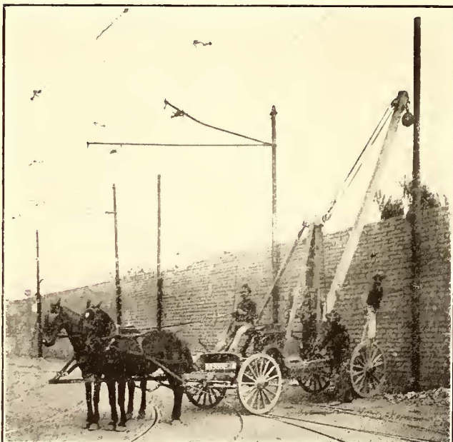
WAGON FOR SETTING POLES
