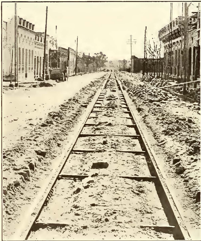
TRACK WORK AT REDUCTO STATION
