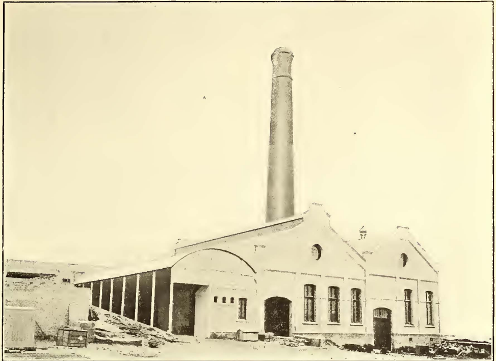
MONTEVIDEO TRAMWAYS POWER HOUSE
