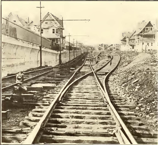
THE WORK IN PROGRESS BETWEEN AVENUES G AND H
