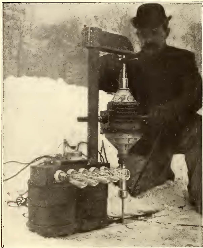
BANK OF LAMPS FOR NIGHT WORK
