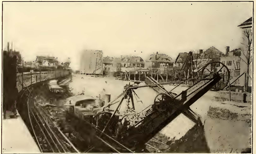
POWER SHOVEL AT WORK ON THE BRIGHTON BEACH LINE
