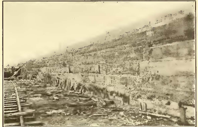
PART OF COMPLETED RETAINING WALL
