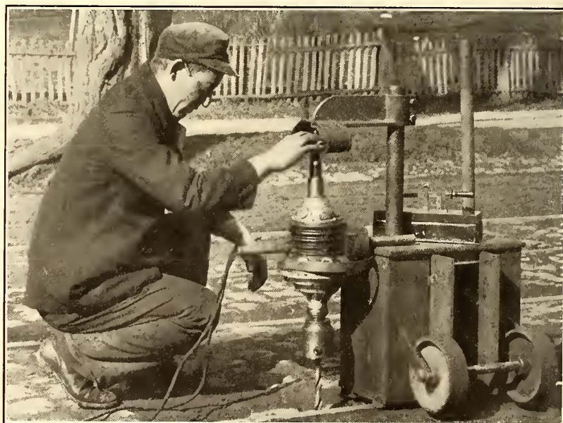
DRILLING A HOLE FOR THE BOND
