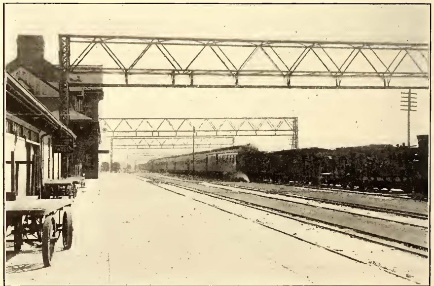
THE TERMINAL YARD, SHOWING BRIDGES FOR CARRYING POWER AND SERVICE WIRES
