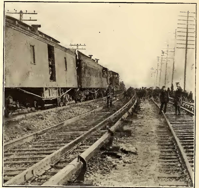
FIGS. 6 AND 7.—TRACK AT WOODLAWN AFTER ACCIDENT, SHOWING EFFECT ON THIRD RAIL
