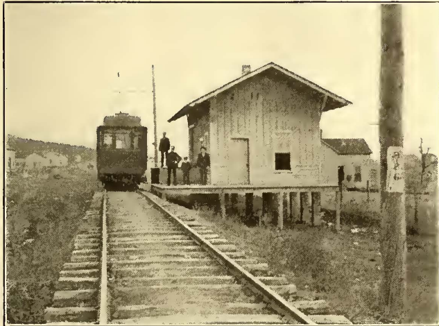
COMBINED FREIGHT AND PASSENGER STATION
