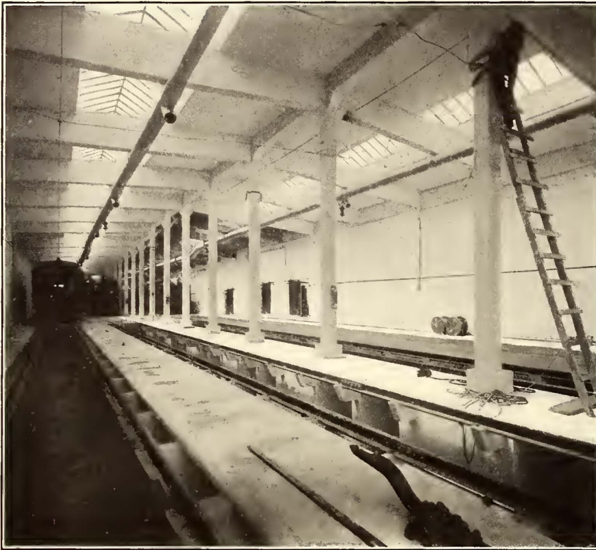
INTERIOR OF THE CAR HOUSE, SHOWING THE CONCRETE ROOF BEAMS, HEATING DUCTS, PITS, ETC.
