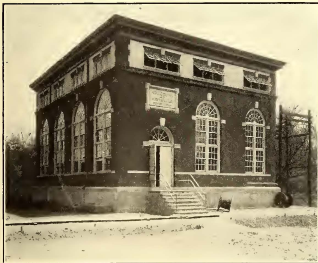
EXTERIOR OF THE ITHAN SUB-STATION
