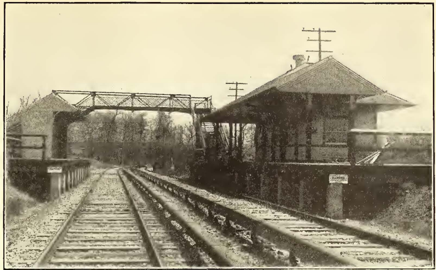
THE VILLA NOVA STATION, WITH TYPICAL FOOT-BRIDGE
