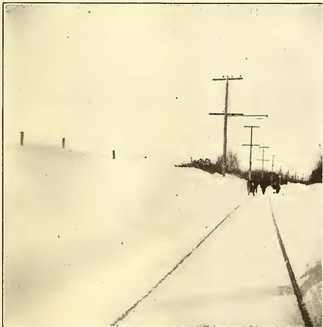
A DRIFT MORE THAN 1000 FT. LONG AND FROM 5 FT. TO 6 FT. HIGH, CLEARED BY PLOW
