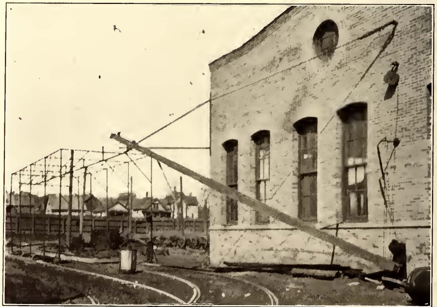
AIR-OPERATED CRANE FOR UNLOADING MATERIAL FROM CARS. A TRANSFER TABLE IS IN THE BACKGROUND
