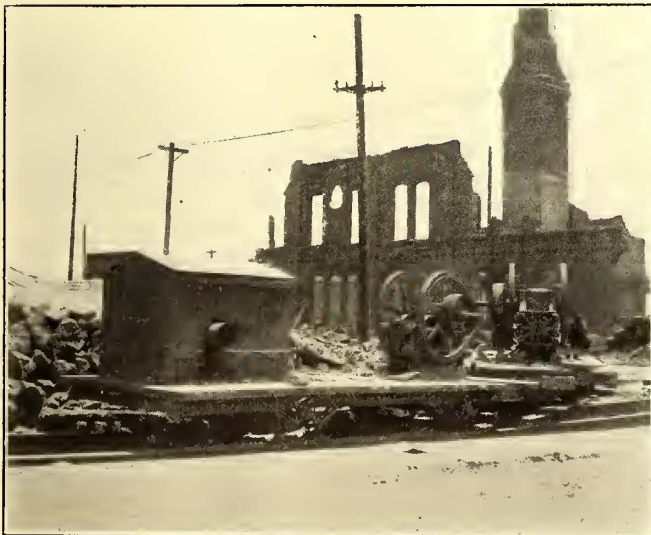
FLAT CAR EQUIPPED WITH CRUSHER FOR BALLASTING
