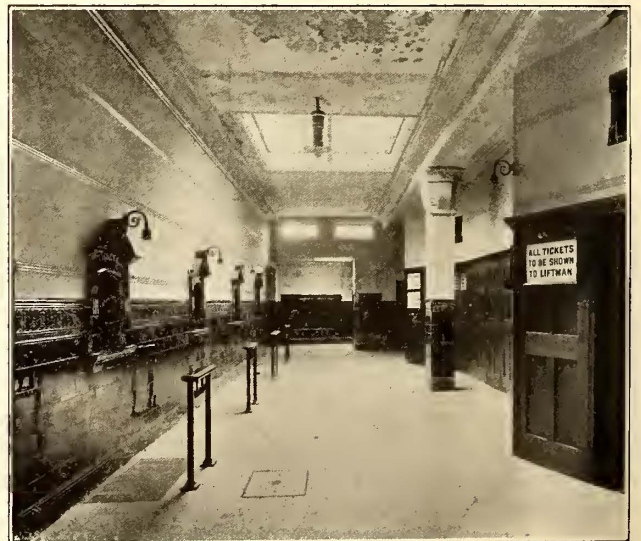
HIGHGATE TICKET OFFICE
