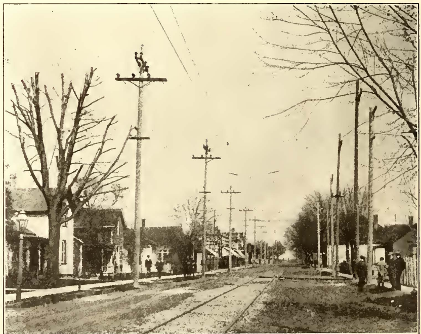
FIG. 15.—CATENARY CONSTRUCTION THROUGH DANVERS
