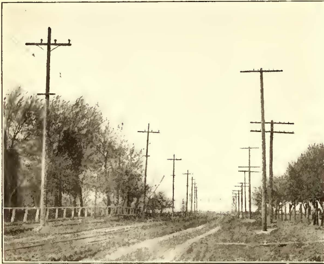
FIG. 14.—VIEW SHOWING SPECIAL CATENARY CONSTRUCTION THROUGH MORTON
