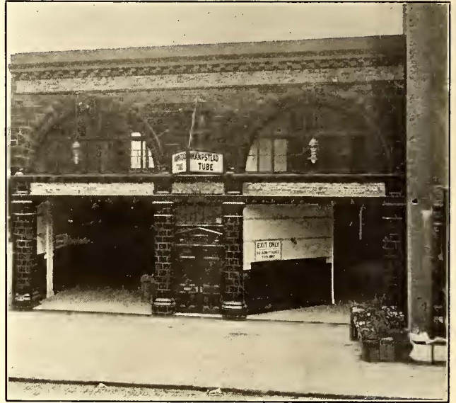
ENTRANCE TO THE HIGHGATE STATION
