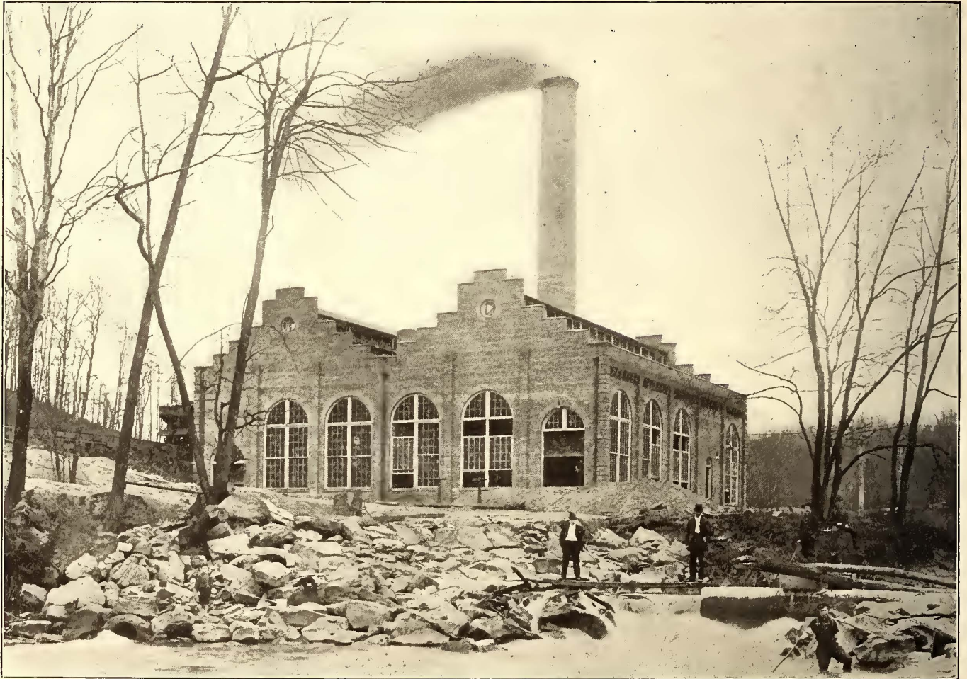
POWER STATION OF PITTSBURG & BUTLER RAILWAY AT RENFREW, SHOWING DAM
