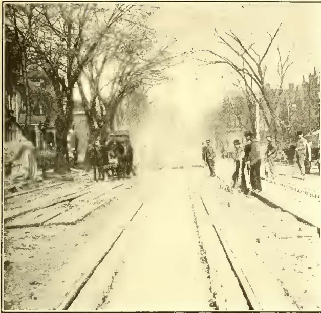
TRACK CONSTRUCTION IN MILWAUKEE STREETS
