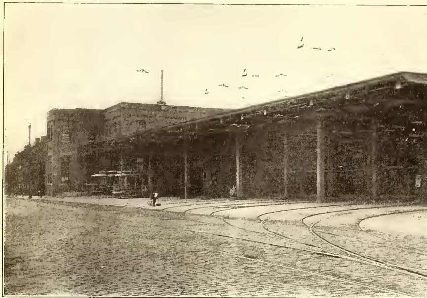
FOURTH AVENUE FRONT OF CAR HOUSE AND SHOPS
