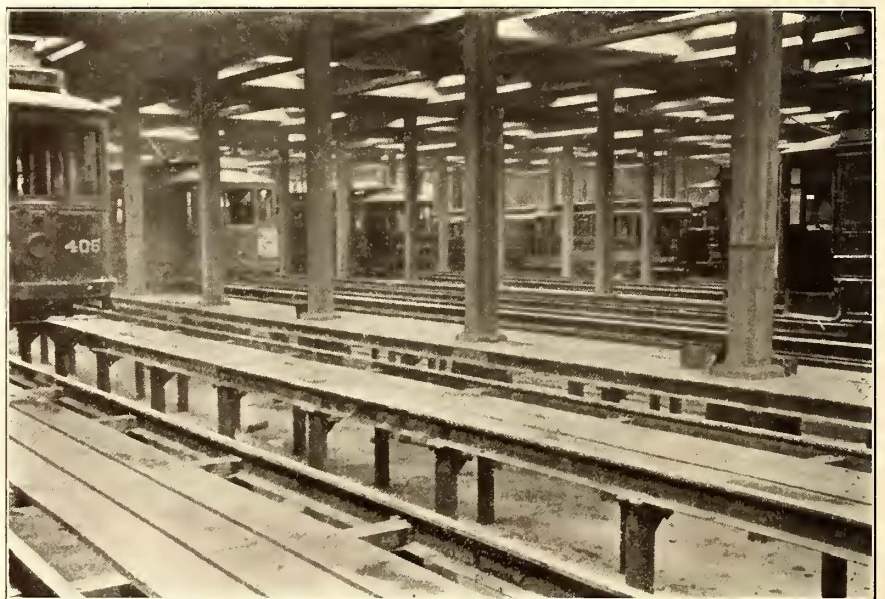
VIEW SHOWING THE OPEN-PIT CONSTRUCTION IN THE NASHVILLE CAR HOUSE
