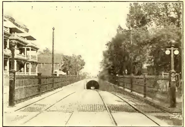
ENTRANCE TO TUNNEL
