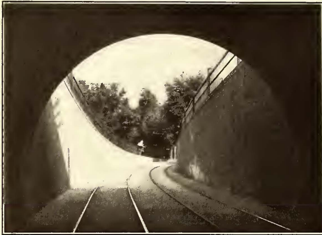
VIEW SHOWING THE RETAINING WALLS
