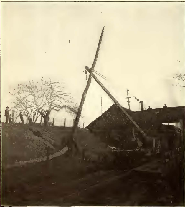
SETTING POLES BY CONSTRUCTION TRAIN
