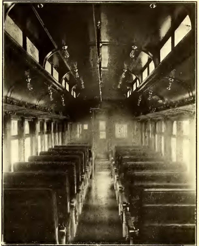
INTERIOR NORTHERN INDIANA RAILWAY CAR
