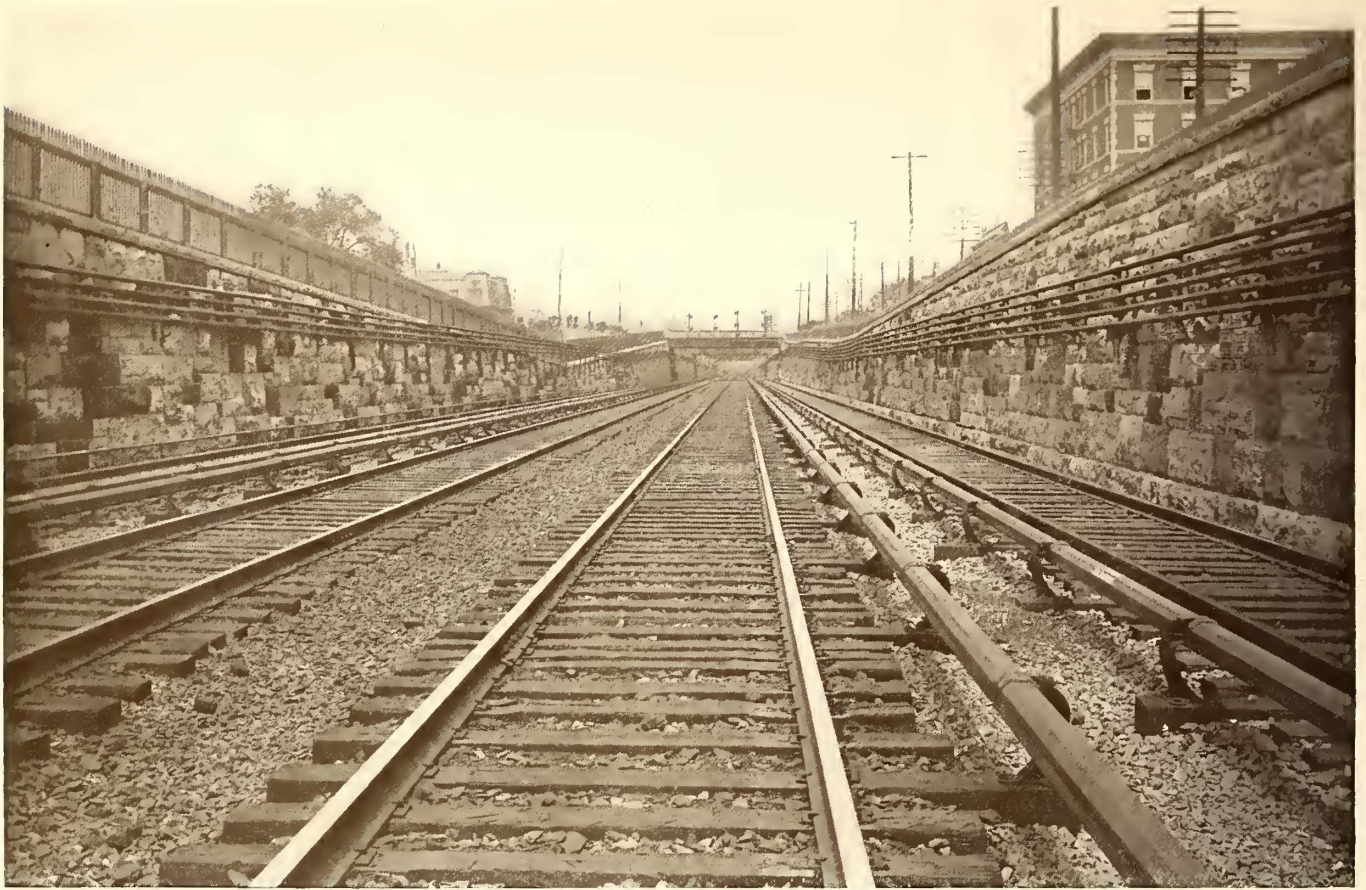
THIRD-RAIL CONSTRUCTION IN HARLEM CUT, NEW YORK CENTRAL RAILROAD
