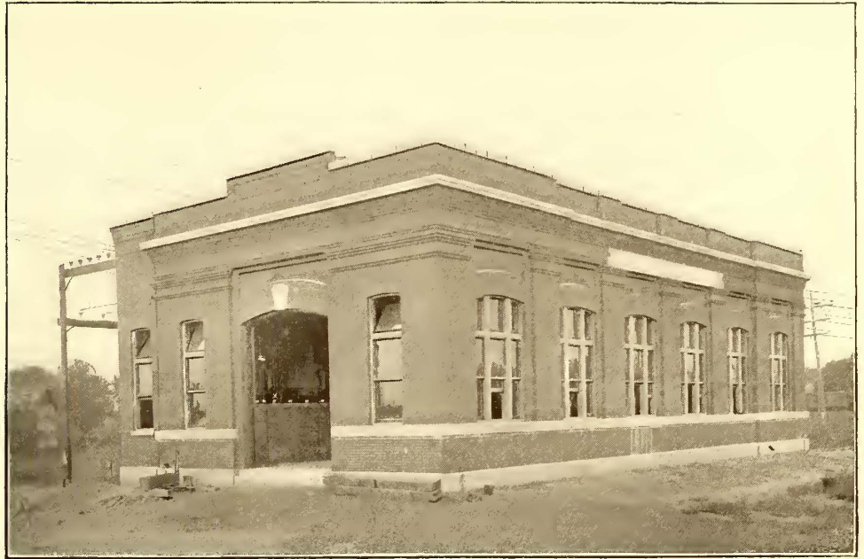
EXTERIOR OF NEWFIELD SUBSTATION, WEST JERSEY & SEASHORE RAILROAD
