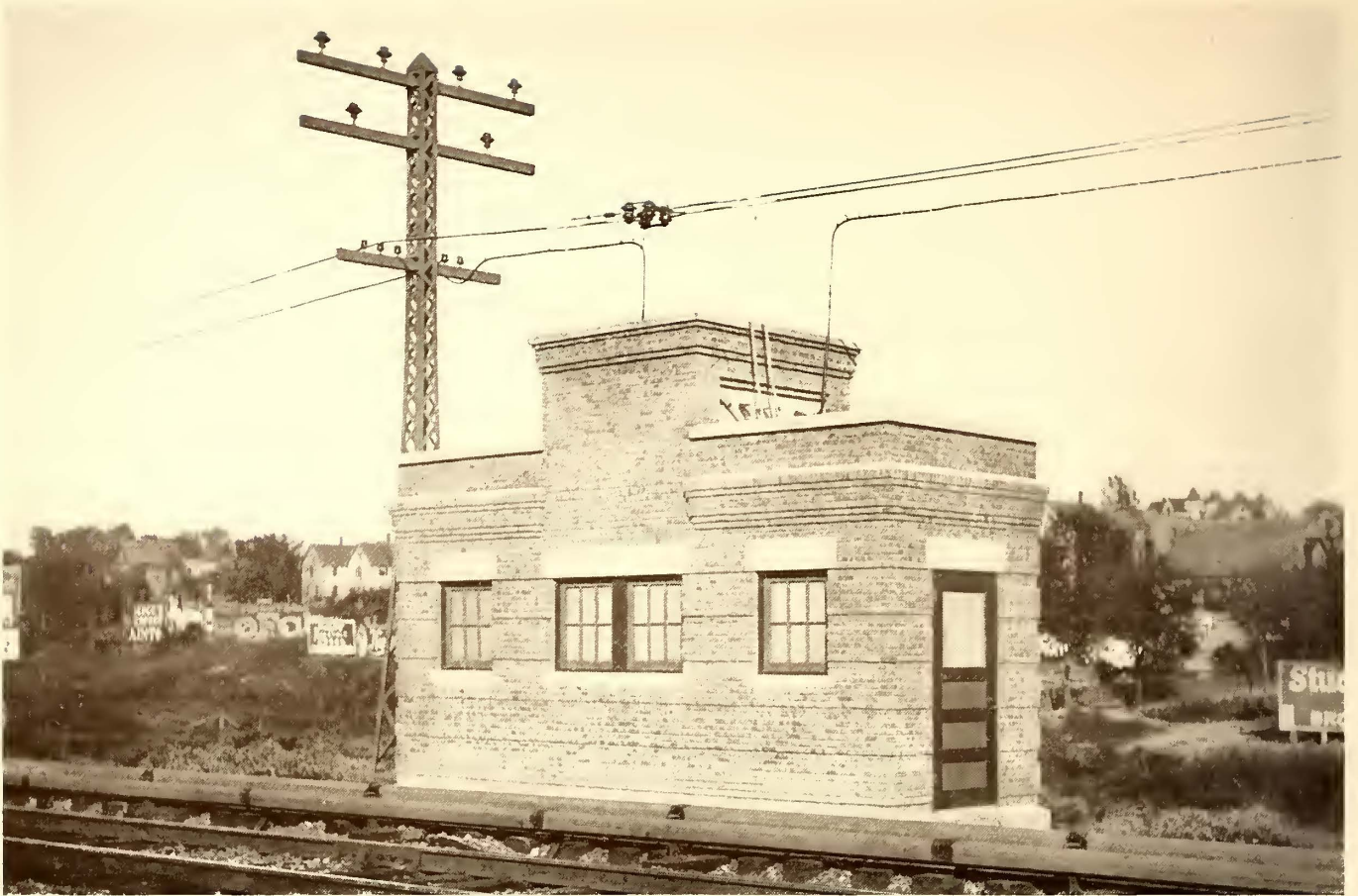
TYPICAL CIRCUIT BREAKER HOUSE, NEW YORK CENTRAL RAILROAD
