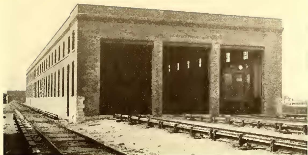
EXTERIOR OF INSPECTION SHED AT ROCKAWAY PARK
