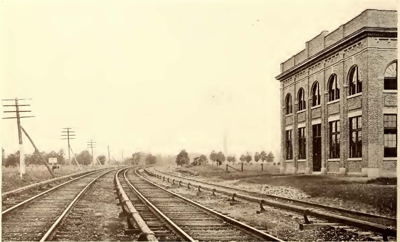
EXTERIOR OF CLARK'S MILLS SUB-STATION, WEST SHORE RAILROAD
