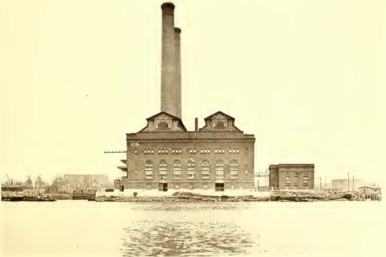
VIEW FROM RIVER OF PORT MORRIS POWER STATION OF NEW YORK CENTRAL RAILROAD, SHOWING RELATION OF POWER STATION AND SWITCH-HOUSE
