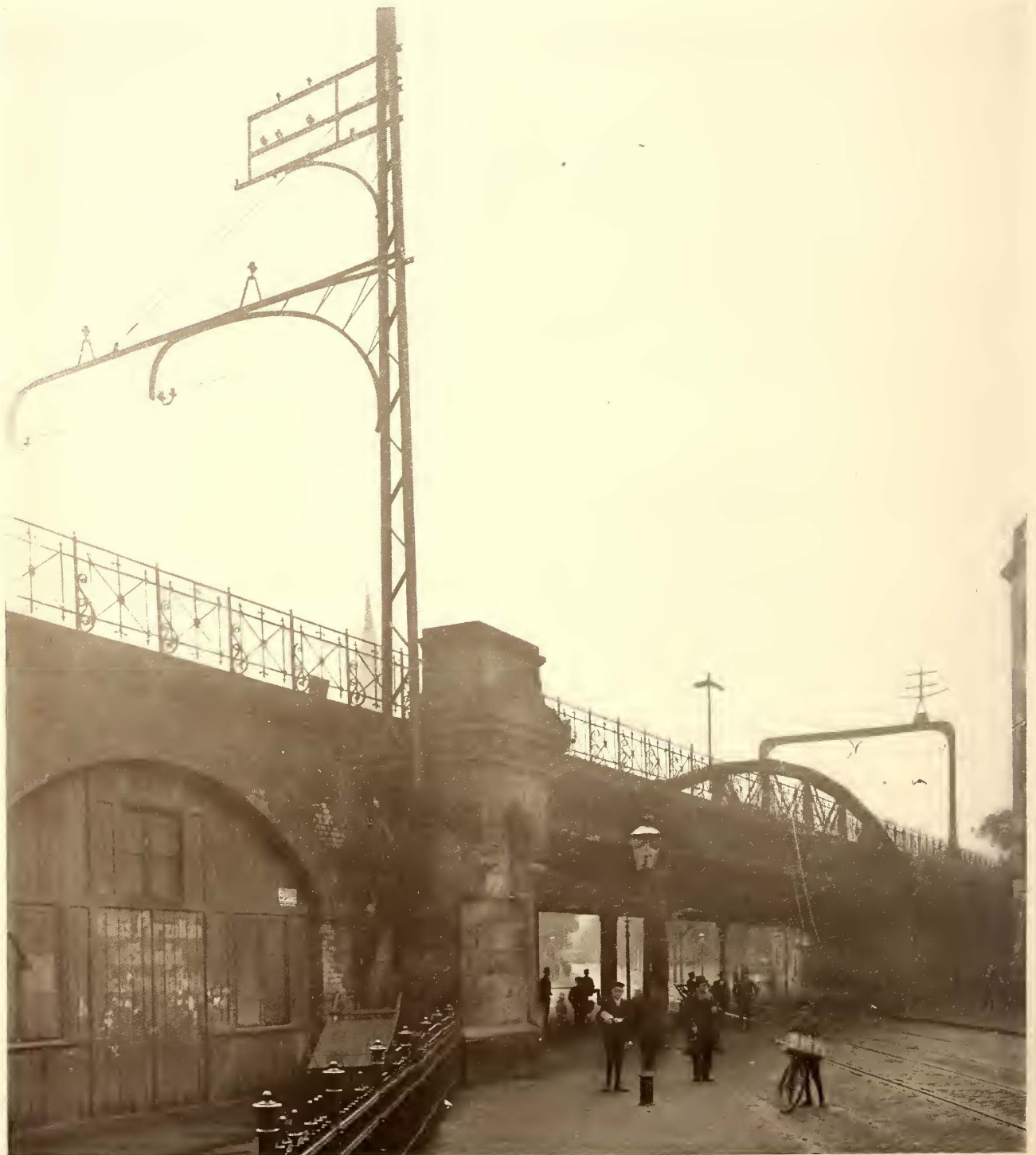
OVERHEAD LINE ON THE HAMBURG-ALTONA RAILWAY, SINGLE-PHASE, 6000 VOLTS, 25 CYCLES
