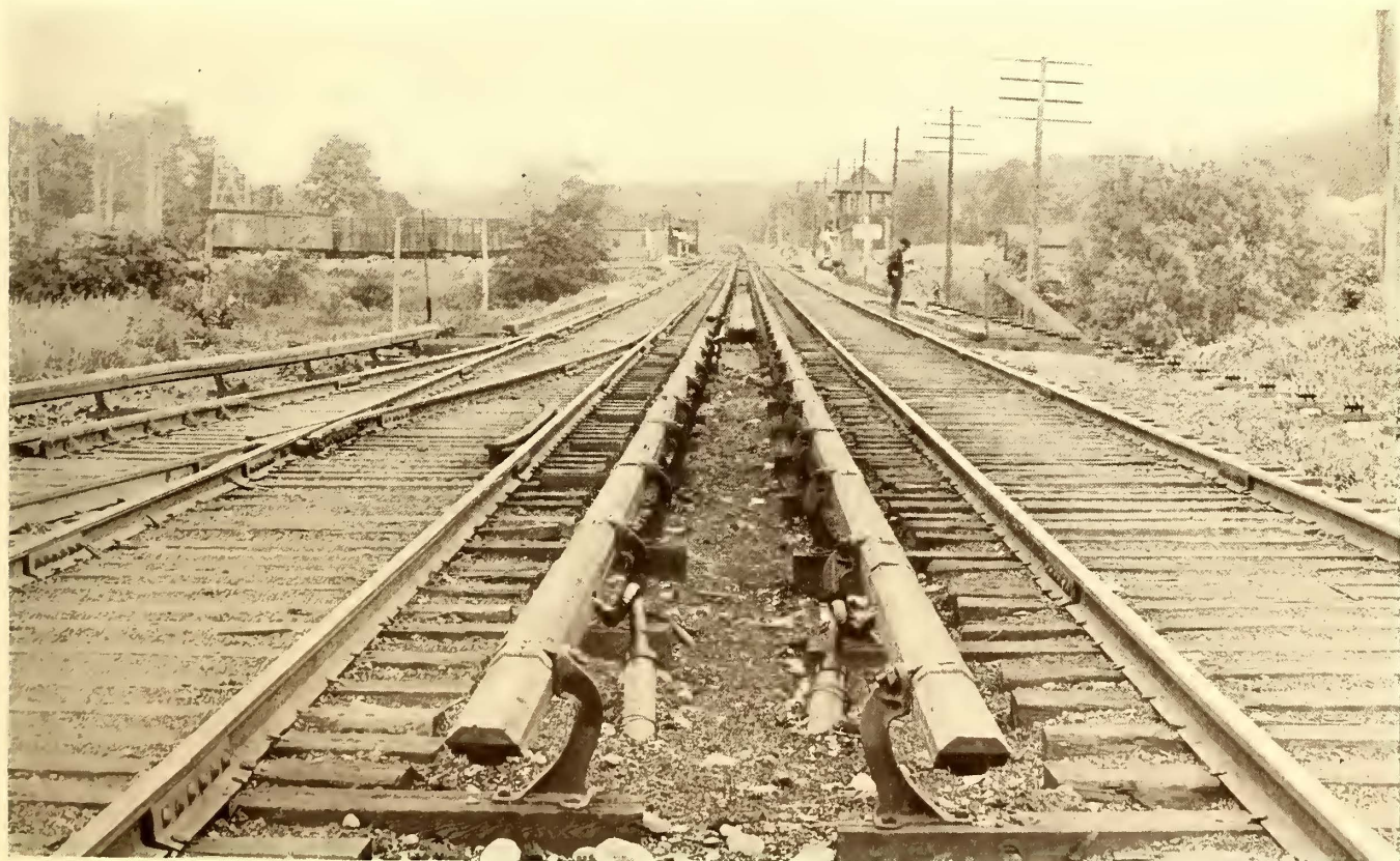
THIRD-RAIL ON TANGENT WITH WOODEN PROTECTION, SHOWING FORM OF JUMPER USED
