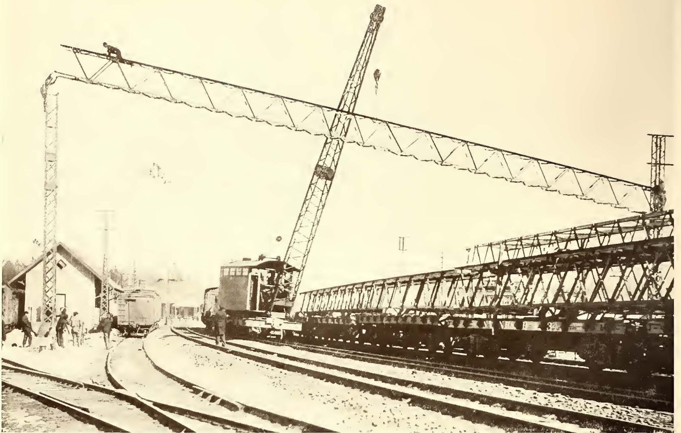
RAISING TOP GIRDER FOR FOUR-TRACK OVERHEAD TROLLEY BRIDGE, NEW HAVEN RAILROAD
