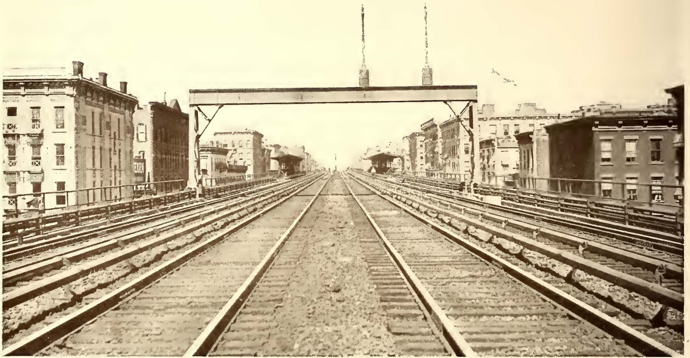
SIGNAL BRIDGE AT 168TH ST., LOOKING NORTH, NEW YORK CENTRAL RAILROAD
