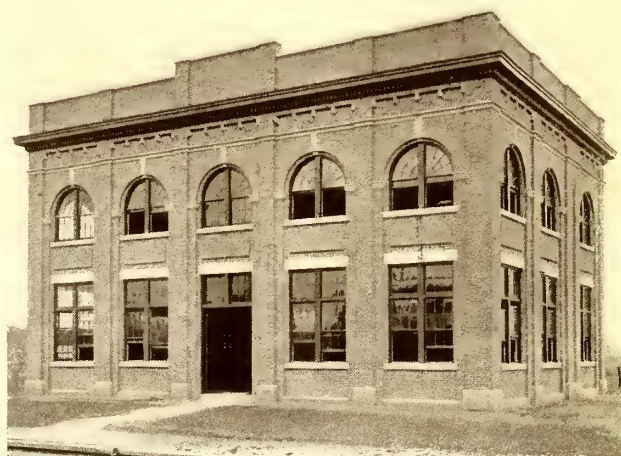
EXTERIOR OF CLARK'S MILLS SUBSTATION
