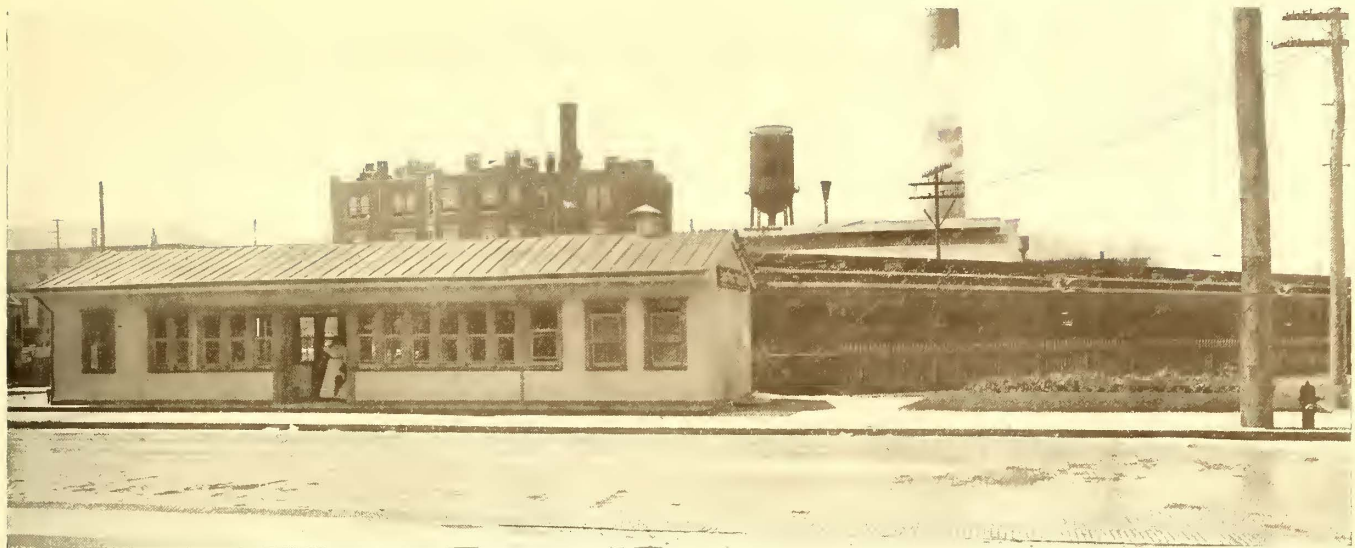
MAIN TERMINAL STATION FOR ELECTRIC CARS OF THE WEST JERSEY & SEASHORE RAILROAD, TENNESSEE AVENUE, ATLANTIC CITY
