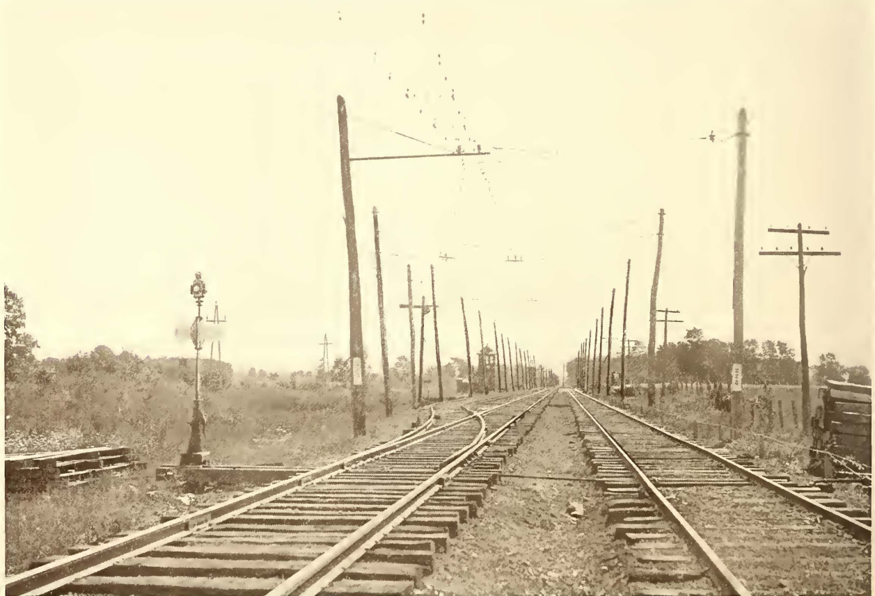
SIDING AT MORTIMER, ERIE RAILROAD, SHOWING OVERHEAD CONSTRUCTION, SWITCH TOWER, SIGNAL AND SWITCH LOCK
