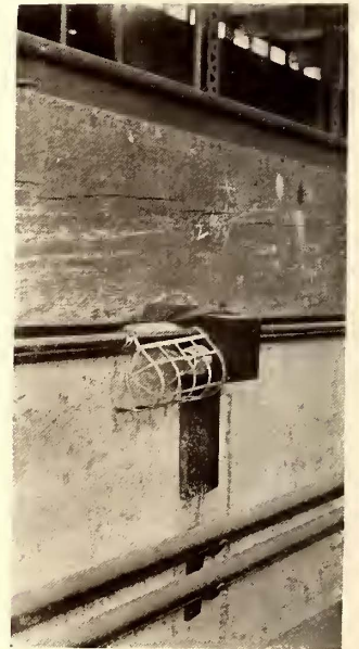
TROLLEY FOR MOVING CARS IN SHED
