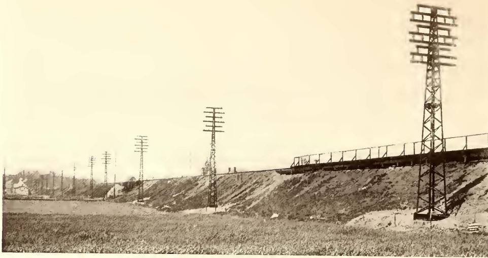
HIGH-TENSION TRANSMISSION LINE BETWEEN LONG ISLAND RAILROAD POWER STATION AND WOODHAVEN JUNCTION
