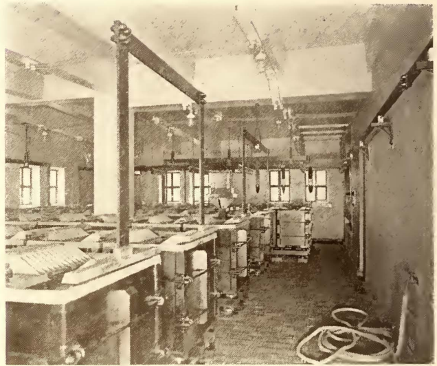
BATTERY ROOM LOOKING SOUTH
