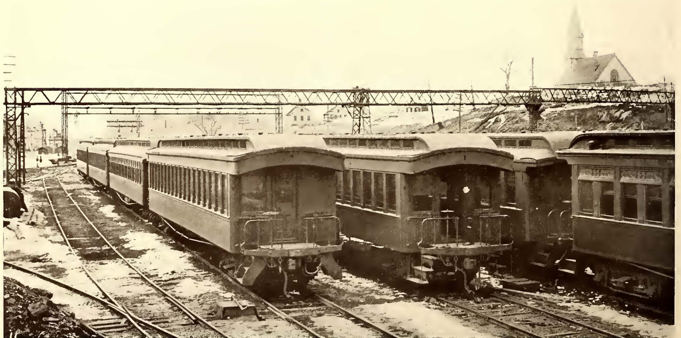
BRIDGES IN YARDS, VIEW TAKEN BEFORE ERECTION OF CATENARY, NEW HAVEN RAILROAD
