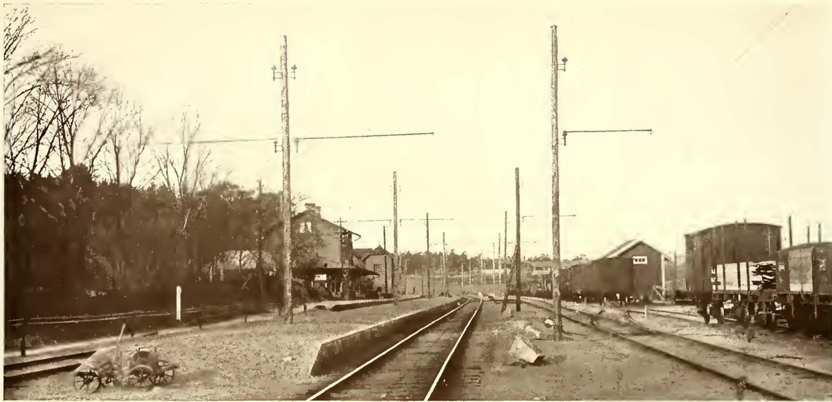
VIEW OF OVERHEAD CONSTRUCTION ON SWEDISH STATE RAILWAYS
