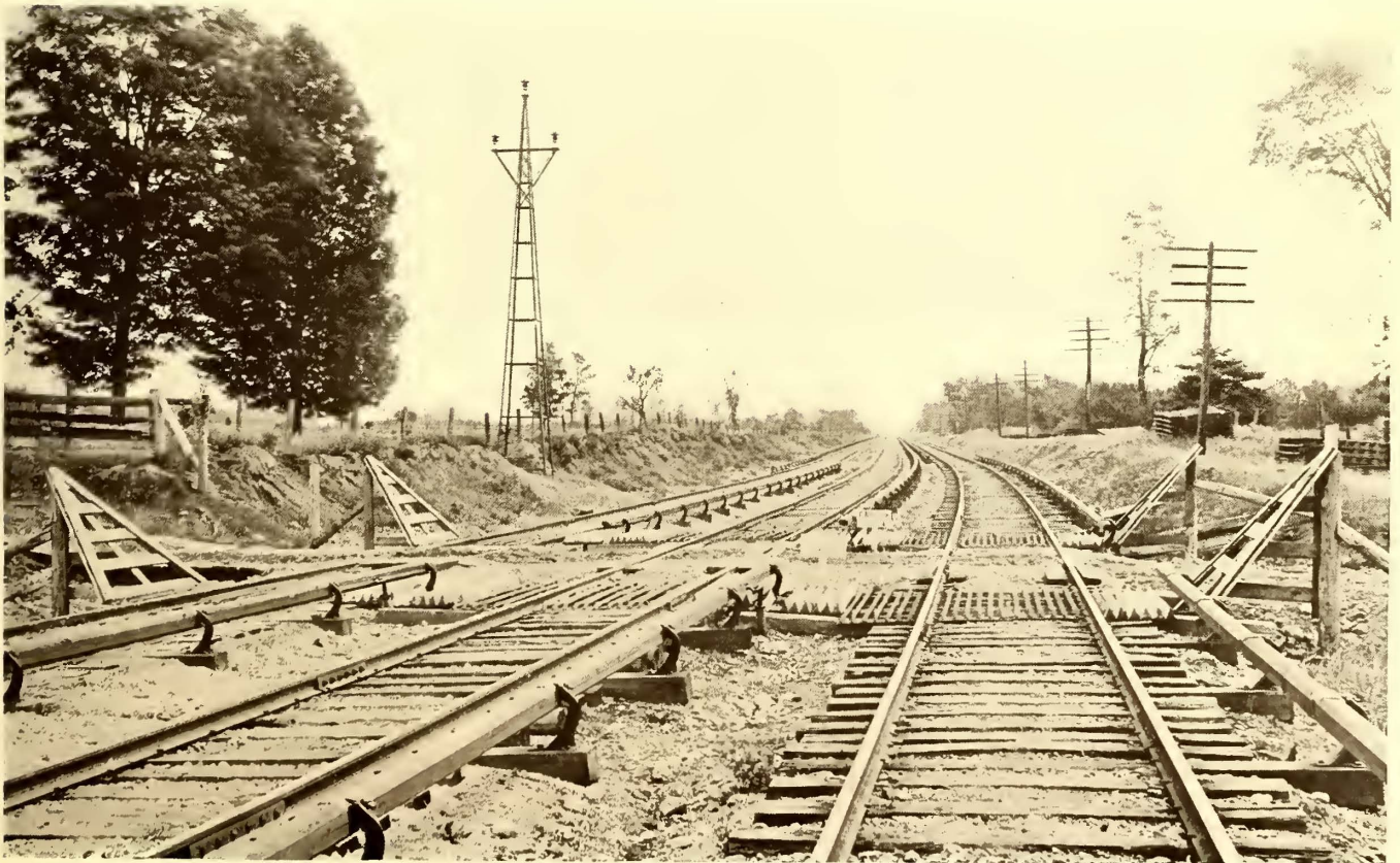
VIEW OF WEST SHORE TRACKS, SHOWING TYPICAL GRADE CROSSING
