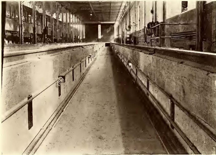
PITS AT DUNTON INSPECTION SHED, SHOWING METHOD OF LIGHTING
