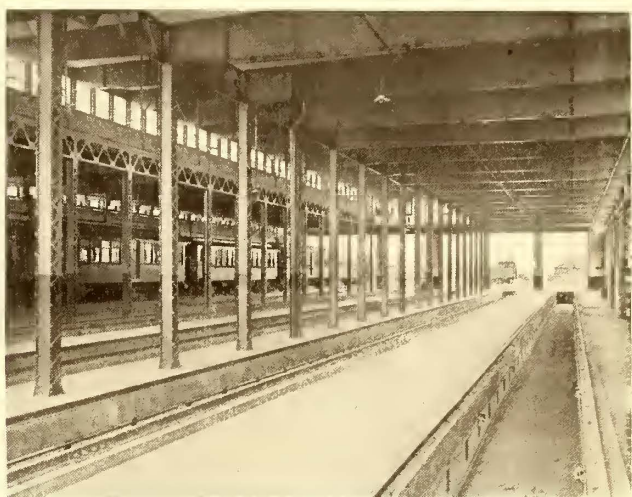
INTERIOR OF DUNTON CAR-HOUSE
