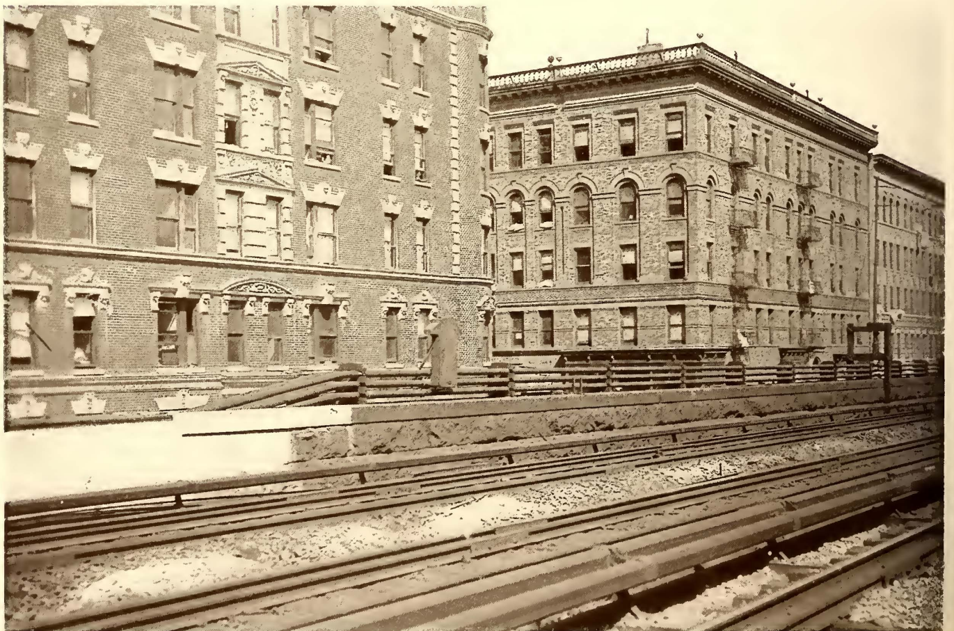
TYPICAL PIPE CONDUIT, LOOKING NORTH FROM 160TH ST., NEW YORK CENTRAL RAILROAD
