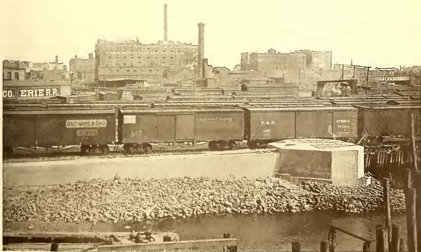
MOTT HAVEN SPlicing CHAMBER AT HARLEM RIVER, NEW YORK CENTRAL RAILROAD
