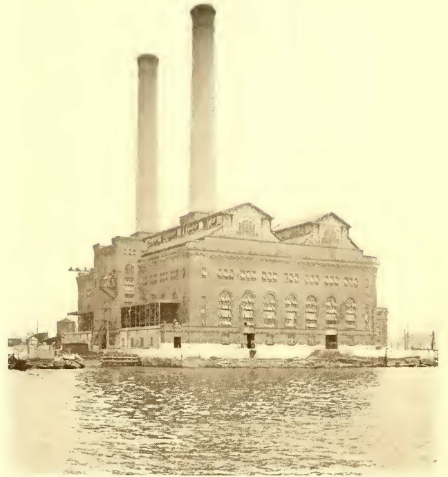
EXTERIOR OF PORT MORRIS POWER STATION
