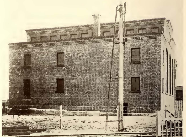
EXTERIOR OF EAST NEW YORK SUBSTATION
