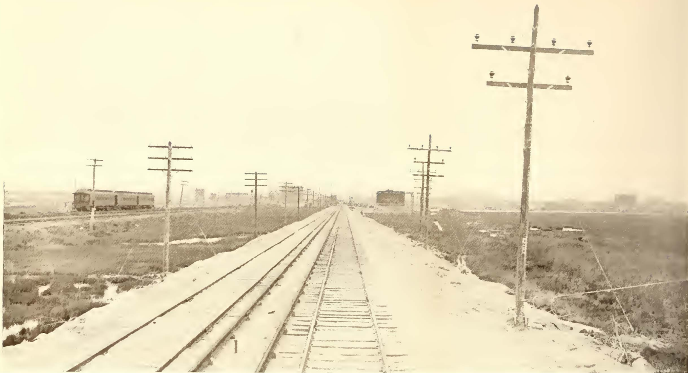
ATLANTIC CITY MEADOWS, LOOKING TOWARD ATLANTIC CITY SUBSTATION, WEST JERSEY & SEASHORE RAILROAD
