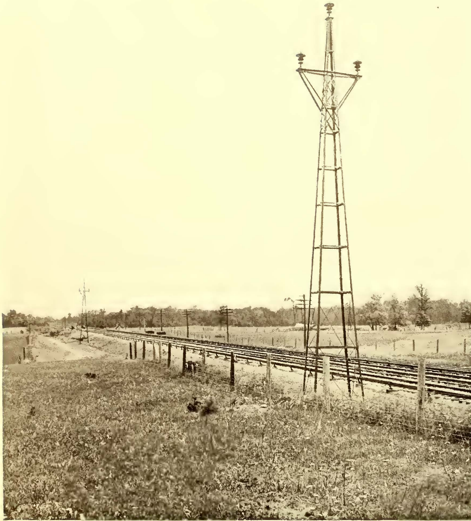
VIEW OF RAILWAY COMPANY'S TRANSMISSION LINE NEAR VERONA, WEST SHORE RAILROAD
