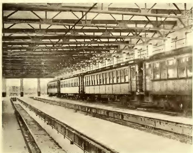
INTERIOR OF INSPECTION SHED AT ROCKAWAY PARK.
