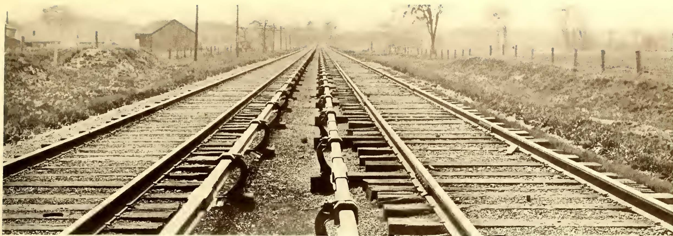
WEST SHORE TRACKS WITH THIRD-RAIL AND FIBRE PROTECTION
