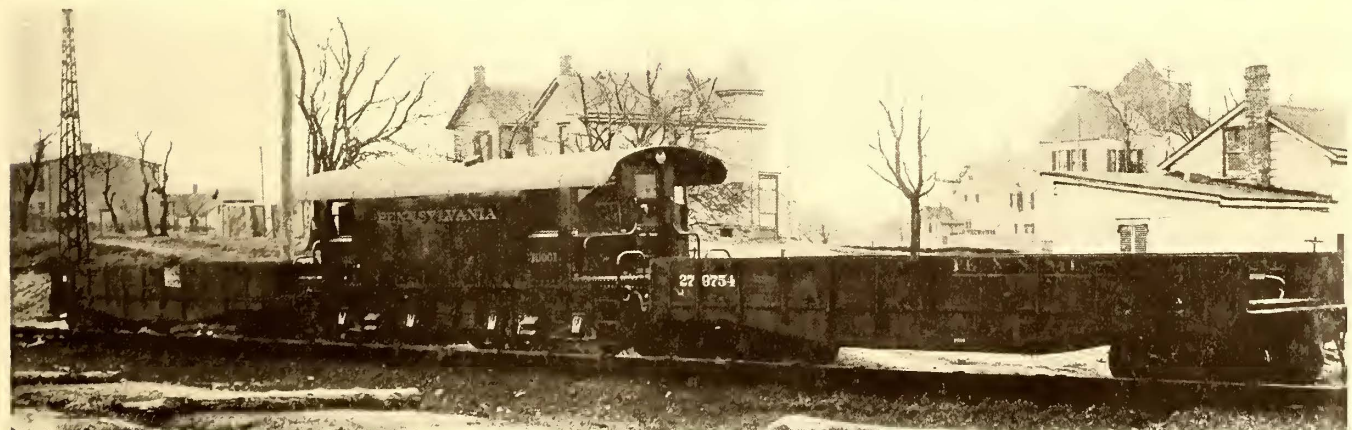
DIRECT-CURRENT LOCOMOTIVE HAULING CONSTRUCTION TRAIN ON LONG ISLAND RAILROAD
