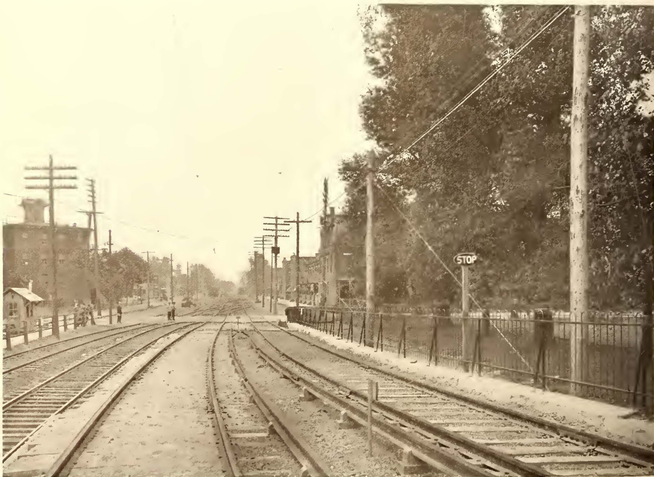
END OF THIRD-RAIL ON TRESTLE AT CAMDEN AND BEGINNING OF TROLLEY, WEST JERSEY & SEASHORE RAILROAD
