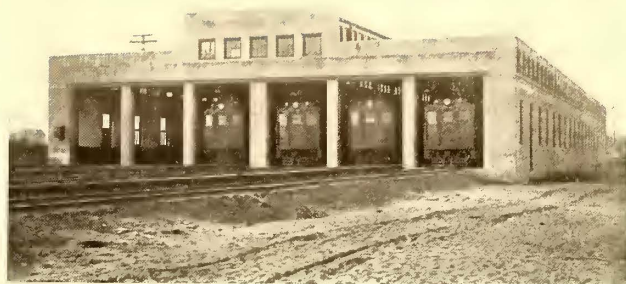
CONCRETE CARHOUSE AT DUNTON
