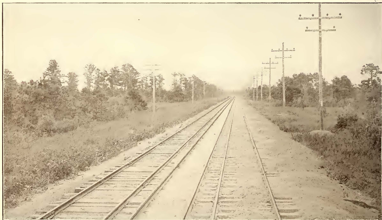
SECTION OF TRACK NEAR MIZPAH, N. J., SHOWING THIRD-RAIL AND TRANSMISSION LINE OF THE WEST JERSEY & SEASHORE RAILROAD
