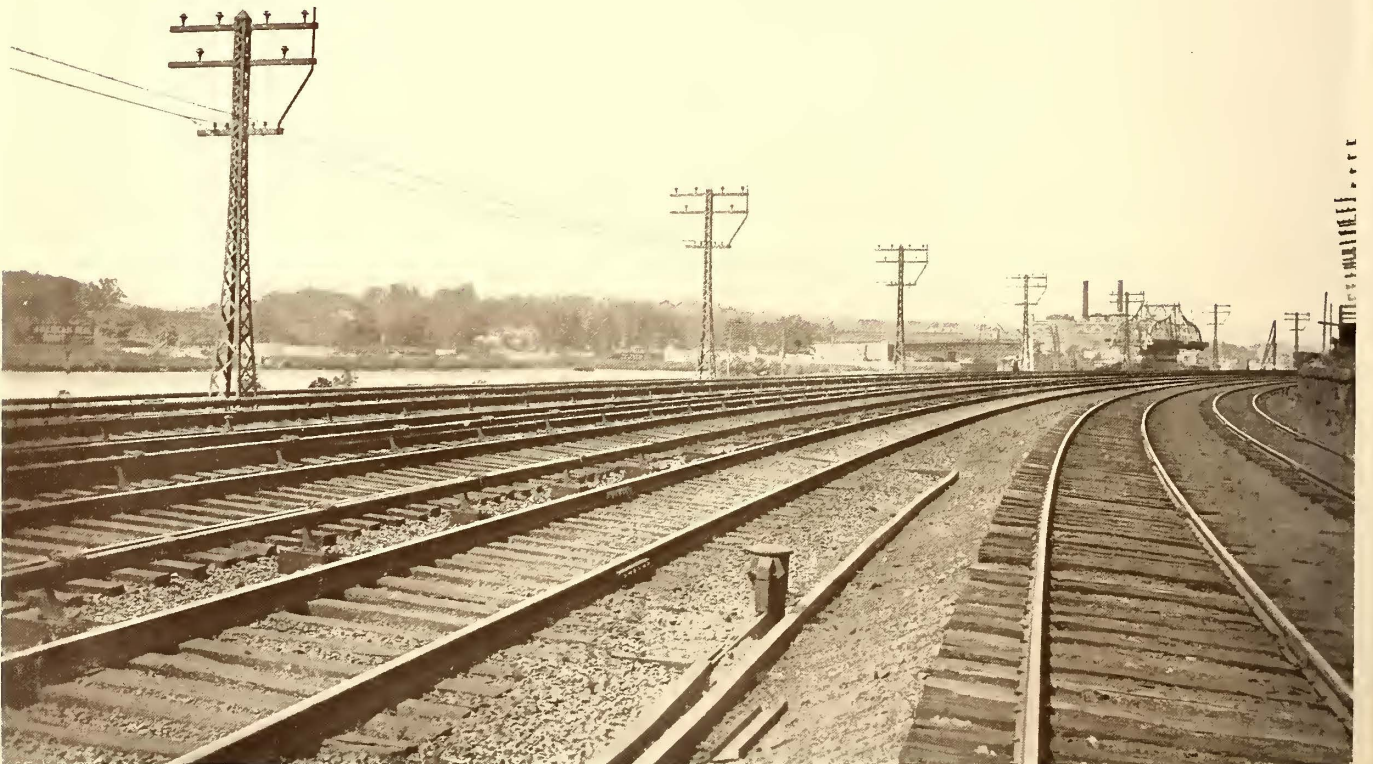
HIGH-TENSION OVERHEAD POLE LINE, HUDSON DIVISION, NEW YORK CENTRAL RAILROAD
