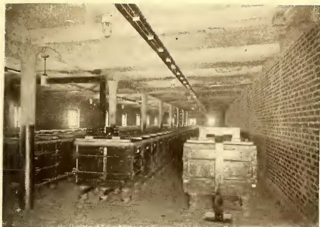
BATTERY ROOM, BRONX PARK SUBSTATION
