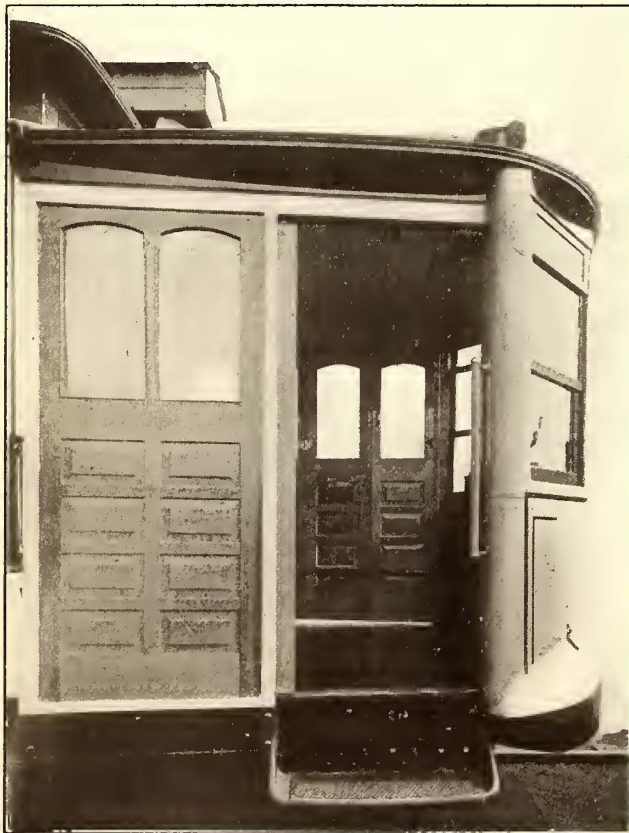
VIEW OF UNOBSTRUCTED EXIT OF MOTORMAN'S PLATFORM WITH ENTRANCE DOOR CLOSED
