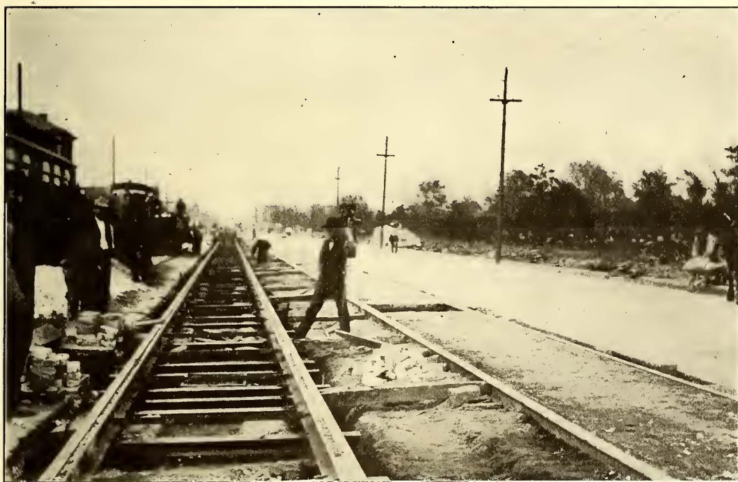
A STRETCH OF TRACK WITH STEEL TIES READY FOR SUBSTRUCTURE
