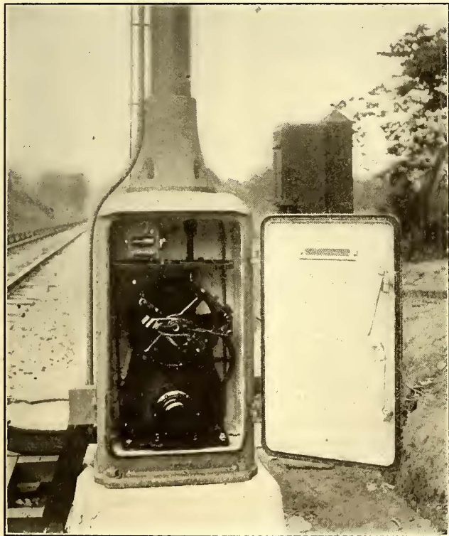
FIG. 6.—SIGNAL MECHANISM EXPOSED
