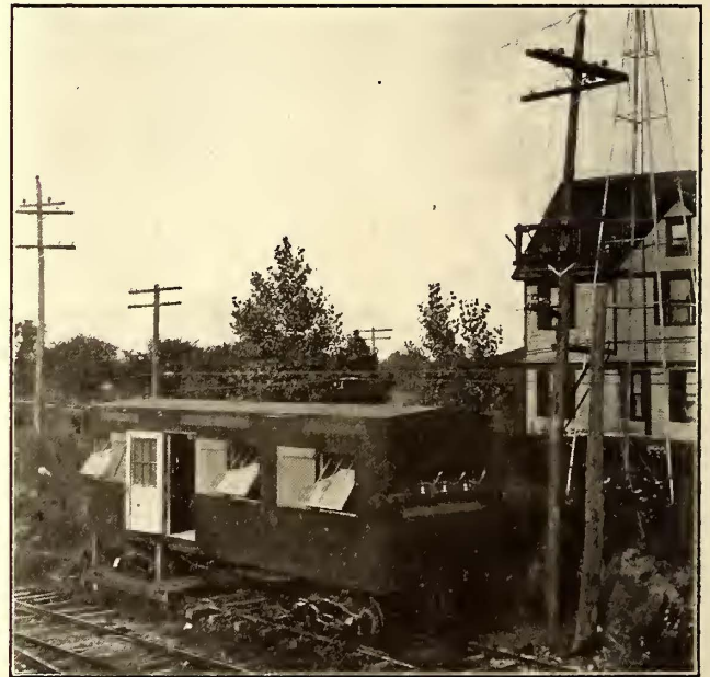
HIGH-TENSION END OF CAR
