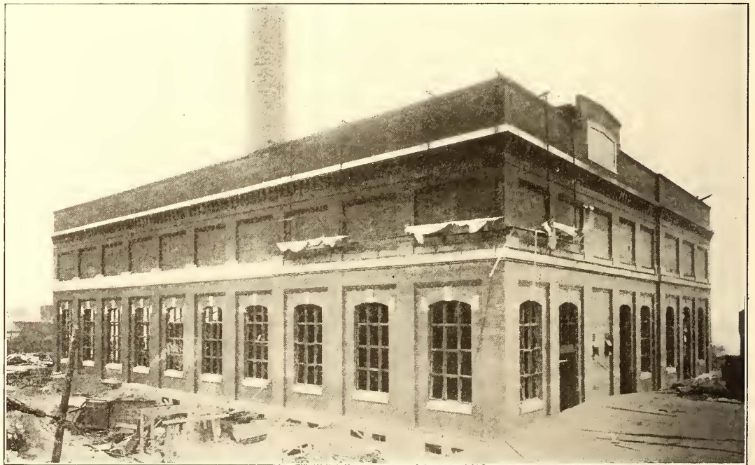
THE HOCHELAGA POWER STATION OF THE MONTREAL STREET RAILWAY COMPANY
