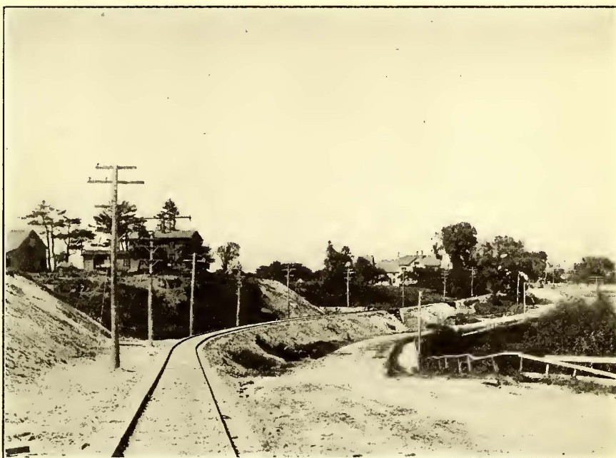
PARALLELING THE HIGHWAY ON AN EMBANKMENT IN WELLS, MAINE
