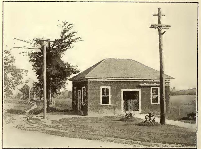
A NEAT SUB-STATION AND WAITING ROOM AT YORK CORNER, MAINE
