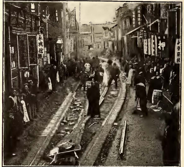
INSTALLING A TURN-OUT IN ONE OF THE MAIN STREETS
