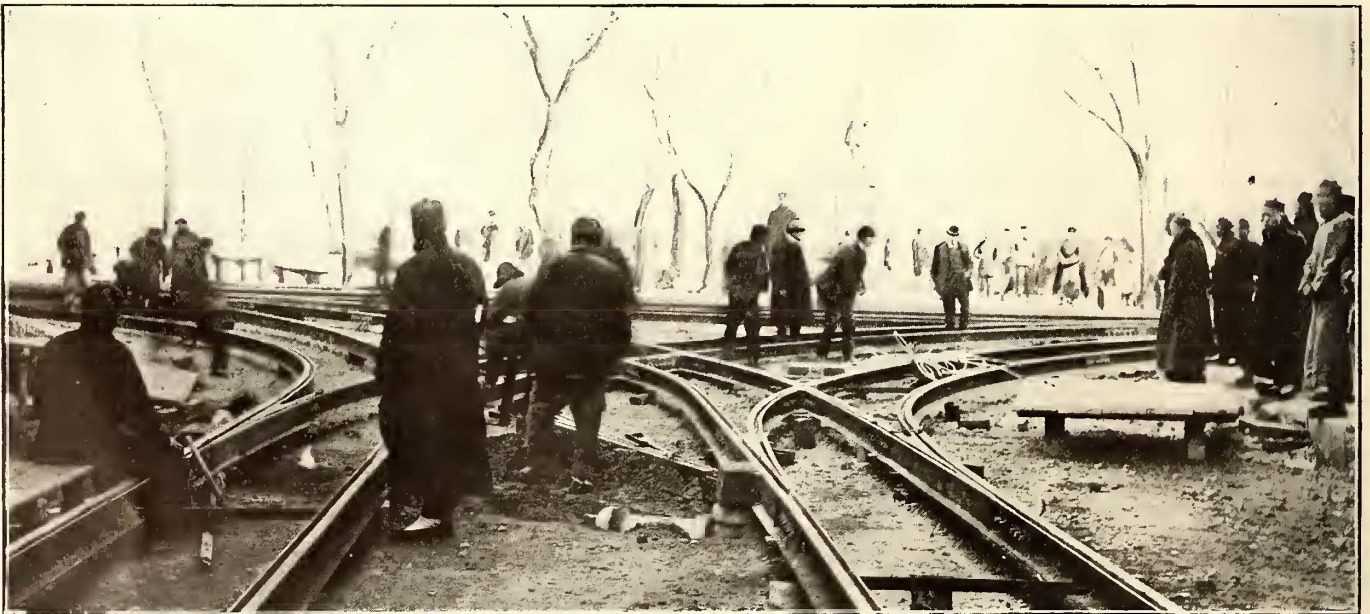
AN INTERESTING PIECE OF SPECIAL WORK BEING INSTALLED BY CHINESE LABORERS
