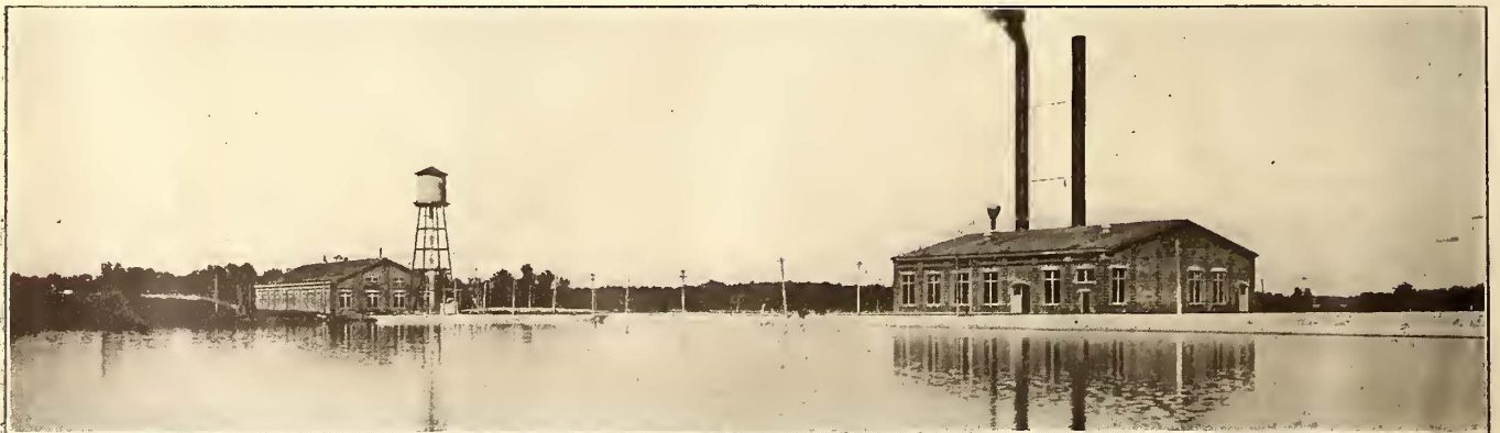
POWER HOUSE, CAR BARN AND ARTIFICIAL LAKE, INDIANAPOLIS & LOUISVILLE LINE
