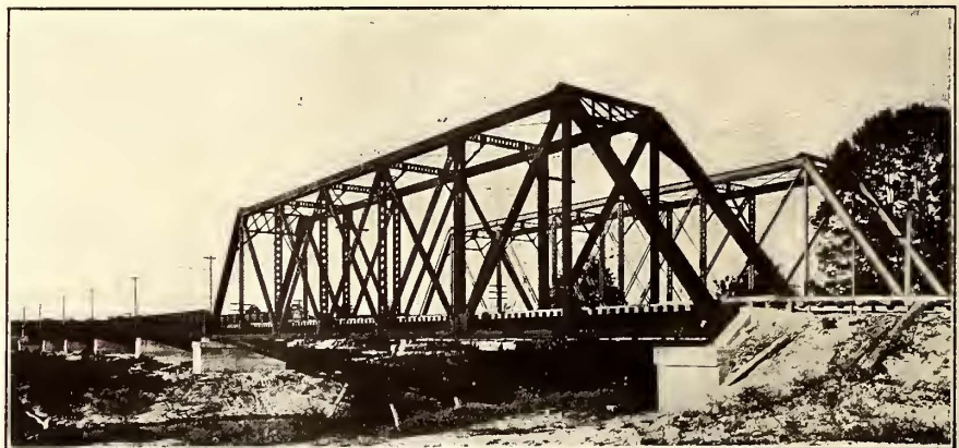
BRIDGE CROSSING THE VERNON FORK OF THE MUSCATATUCK RIVER
