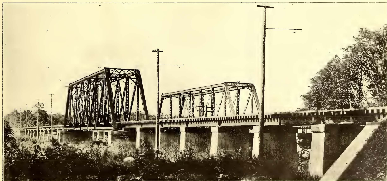
525-FT. BRIDGE ON INDIANAPOLIS & LOUISVILLE LINE, CROSSING MUSCATATUCK RIVER
