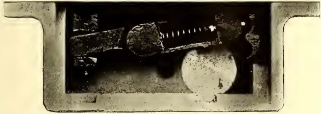
SPRING LOCK FOR TONGUE SWITCH
