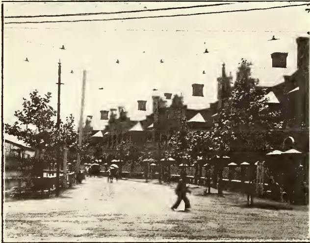
A VIEW OF THE LINE IN THE RESIDENTIAL DISTRICT
