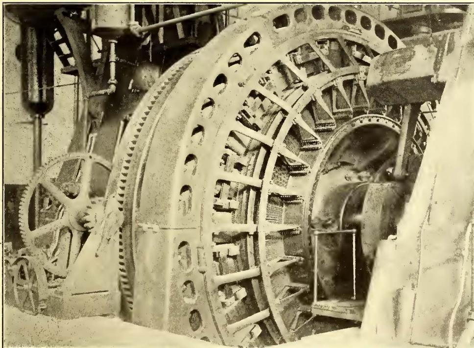
2700-KW COMMUTATING POLE GENERATOR INSTALLED IN BOSTON
