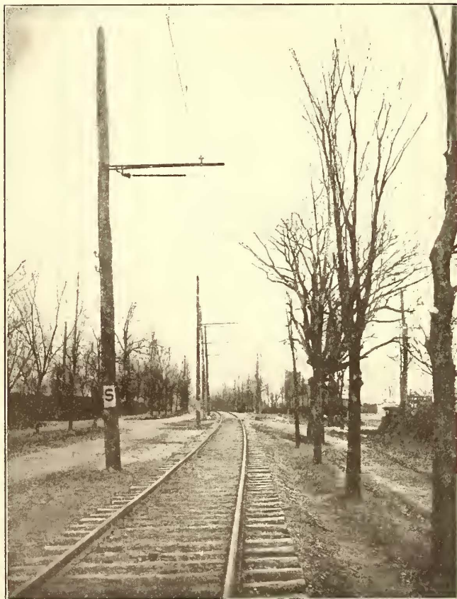
FIG. 19.—CATENARY CONSTRUCTION, SHOWING STEADY BRACES
