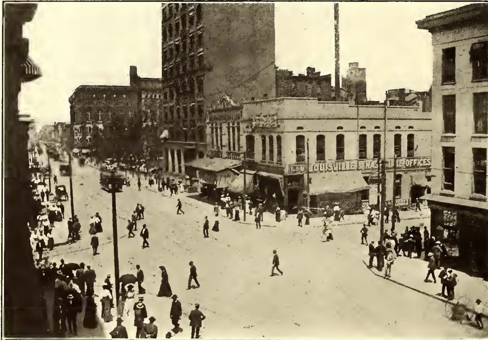
GENERAL VIEW OF FINISHED WORK AT MAIN AND MADISON STREETS, MEMPHIS
