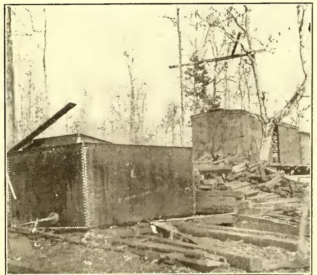
FIG. 3.—DOUBLE TANK USED BY THE SOUTHERN POWER COMPANY. THE OUTSIDE TANK CONTAINS STEAM-HEATED WATER
