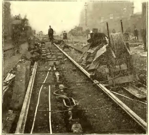
PUTTING IN THE CABLE
