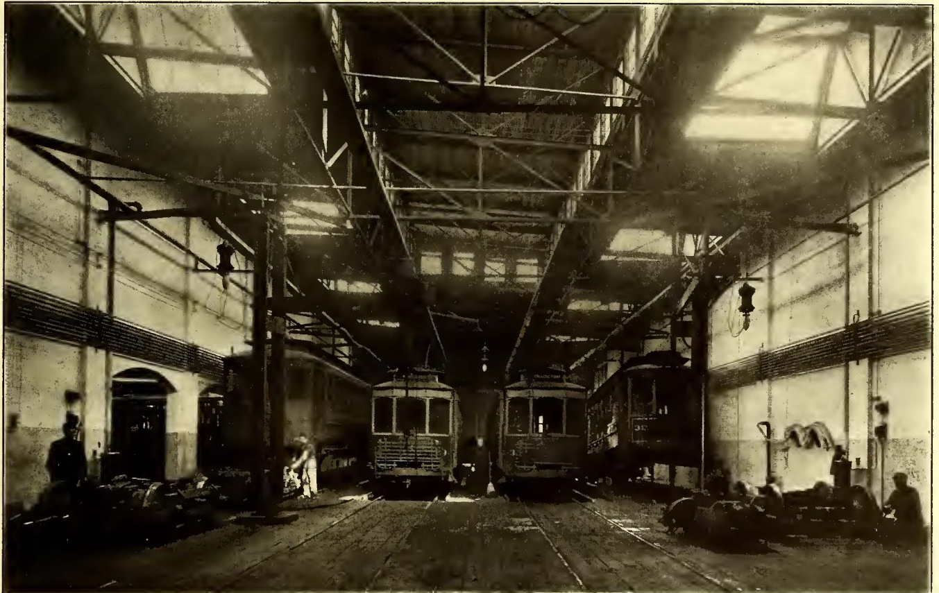
LOOKING TOWARD THE OVERHAULING TRACKS, SHOWING THE LOCATION OF FOUR PNEUMATIC JIB CRANES AND THE METHOD OF RAISING CARS
