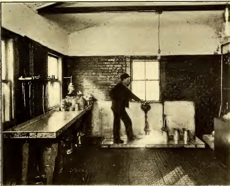
INTERIOR OF OIL HOUSE AT 159TH STREET INSPECTION SHOP
