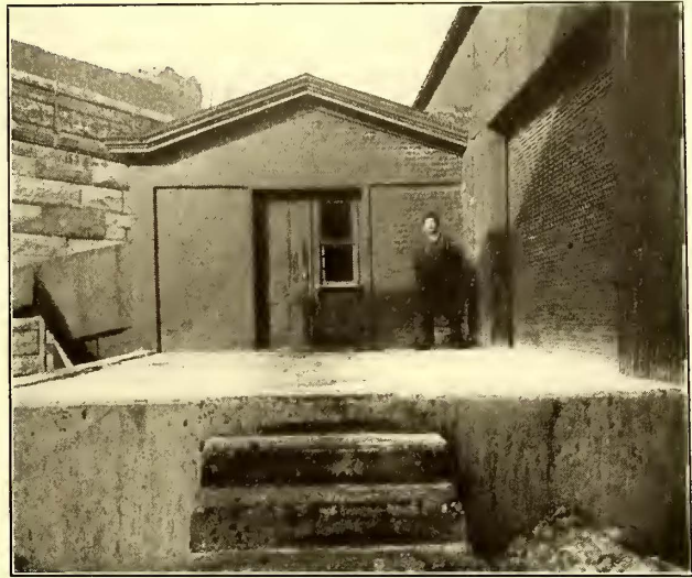
OIL HOUSE AND LOADING PLATFORM AT 159TH STREET INSPECTION SHOP
