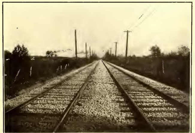
RALEIGH SPRINGS LINE, LOOKING EAST FROM TREGEWANT AVENUE TOWARD BINGHAMPTON, TENN.
