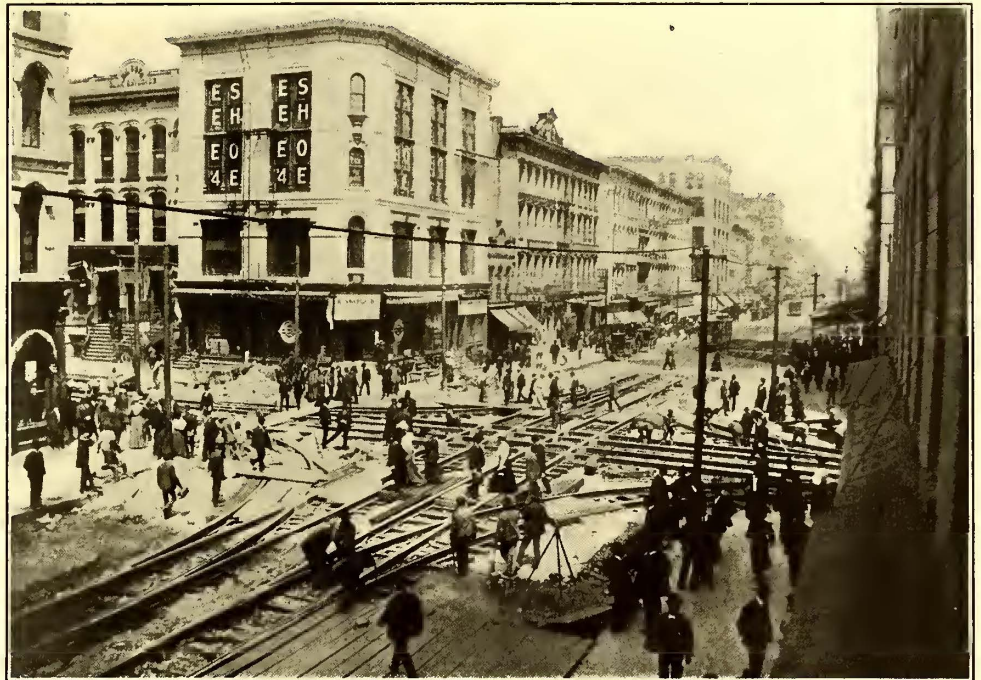
SPECIAL WORK INSTALLATION AT MAIN AND MADISON STREETS, MEMPHIS
