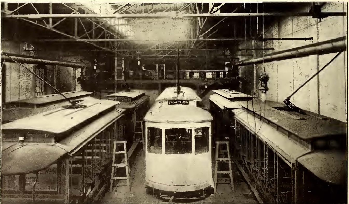
IN THE PAINT SHOP LOOKING TOWARD THE STEEL AND CONCRETE GALLERY
