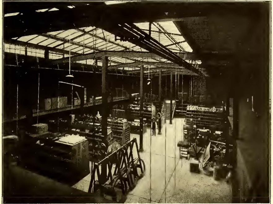
FIG. 11.—INTERIOR OF STOREROOM
