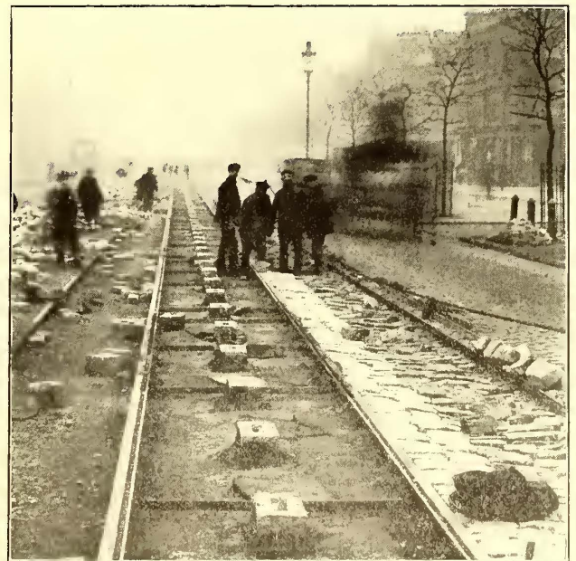
BEGINNING THE WORK OF PAVING
