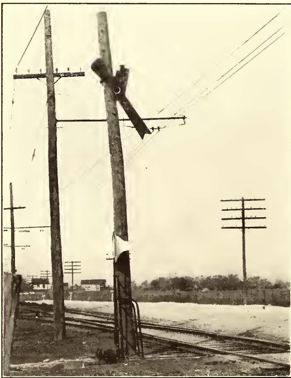
HOME-MADE SEMAPHORE SWITCH SIGNAL
