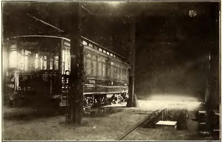
FIG. 13.—TRUCK-CHANGING PITS IN THE BLACKSMITH SHOP
