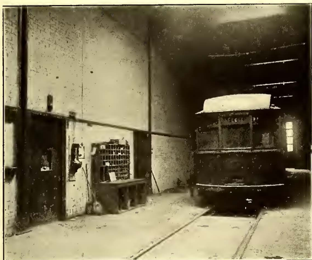
GENERAL INSPECTION ROOM AND CABINET FOR NIGHT FORCE
