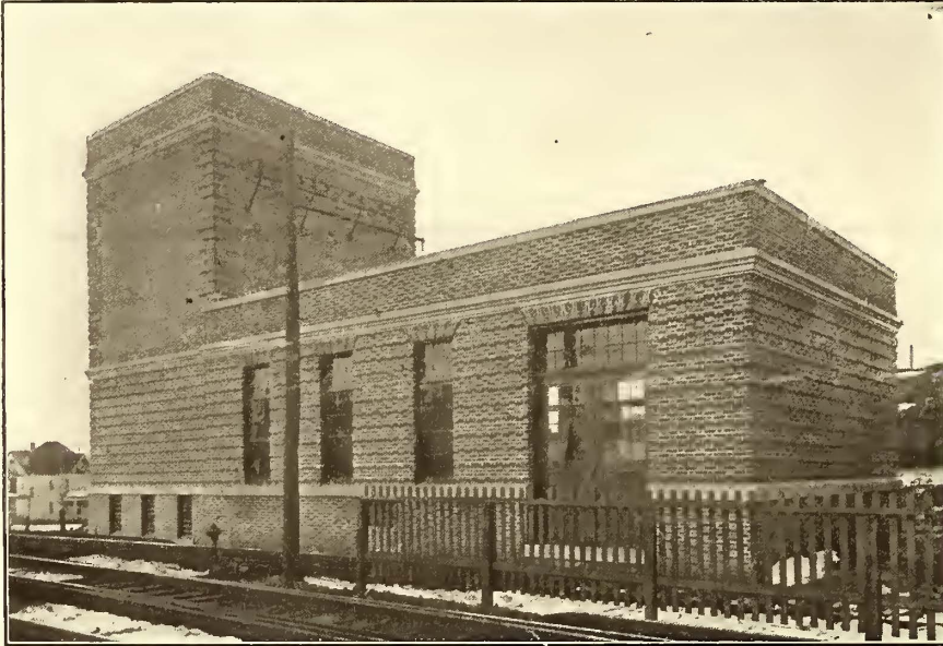
FRONT VIEW OF AVOCA SUBSTATION, SHOWING RUSTICATED BRICK
