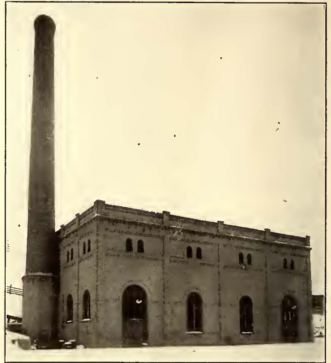
THE JAYENN POWER STATION OF THE FAIRMONT & CLARKSBURG TRACTION COMPANY
