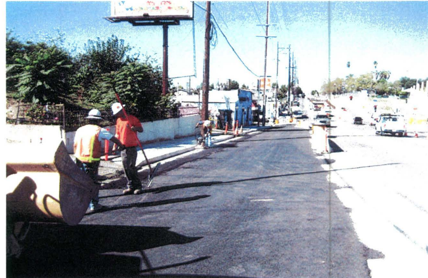
1 st Street – South side view to Lorena Street
