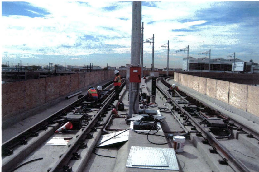
View of LRT bridge guideway looking southwest towards Alameda Street.
