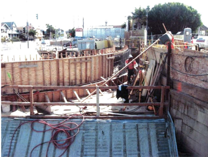
Soto Station - Southwest corner of 1st/Soto where the station entrance is being constructed on the plaza level.
