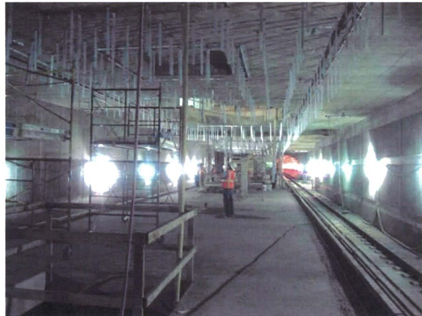
Soto Station – Interior work in the underground rooms progresses as work on the surface structures continues.
