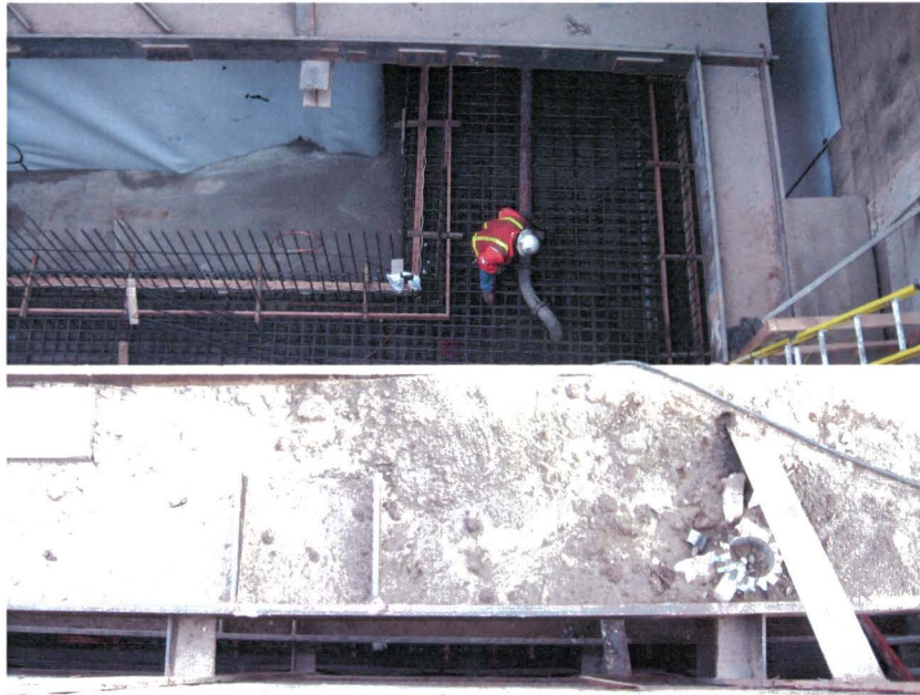
Boyle Heights/Mariachi Plaza Station Emergency Exit
