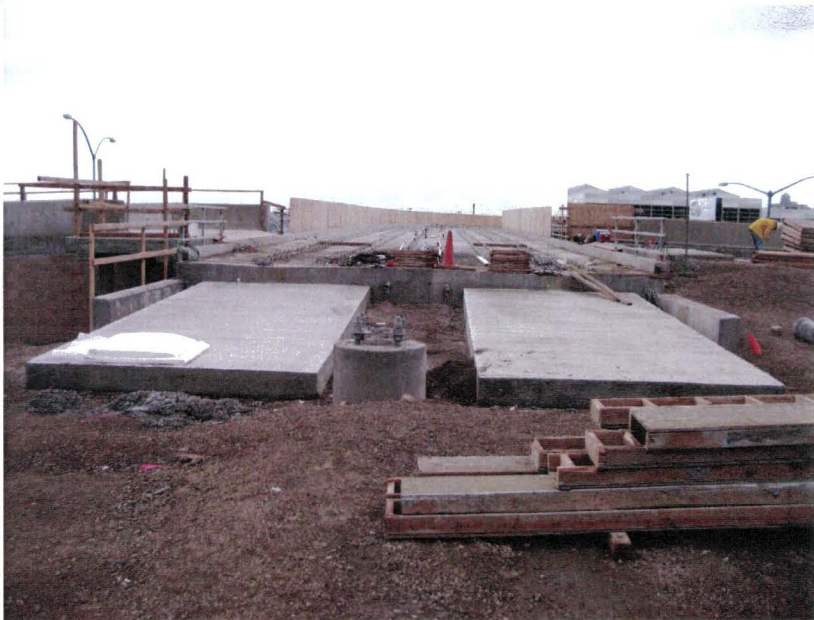
US 101 Freeway LRT Bridge
