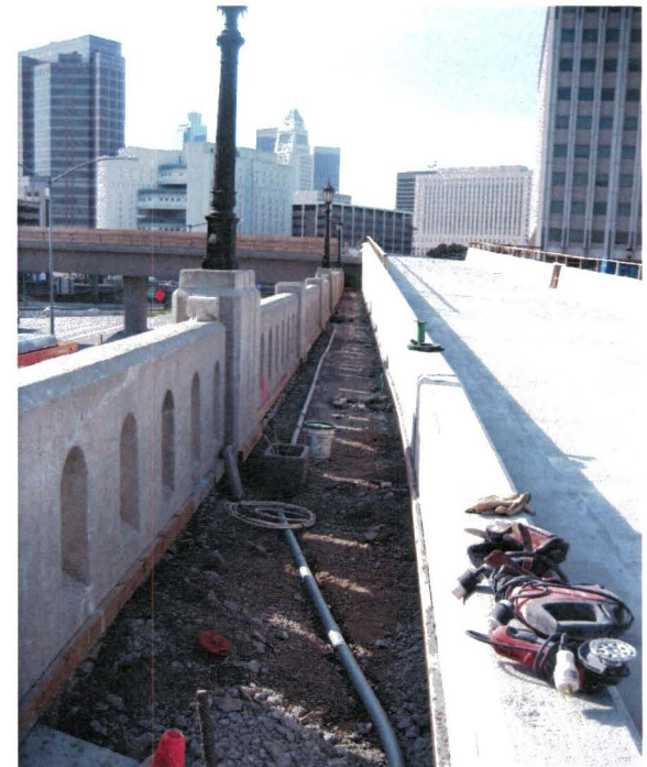
Union Station Baggage Handling Road
