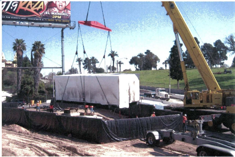
Traction Power Sub-Station 4 Installation
